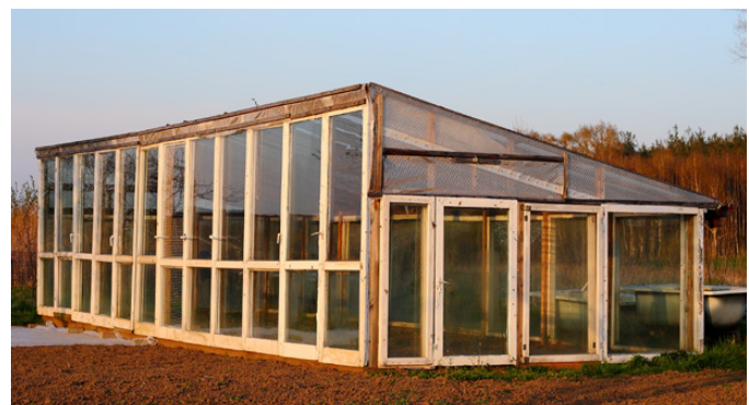
FIG. 3 Greenhouse built from recycled materials.
