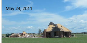
All Photos of Storm By: Larry Weatherford
