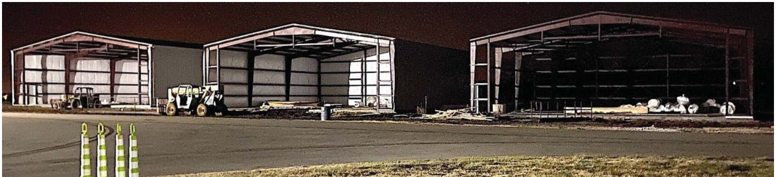
South Grand Lake Regional Airport hangar project.
