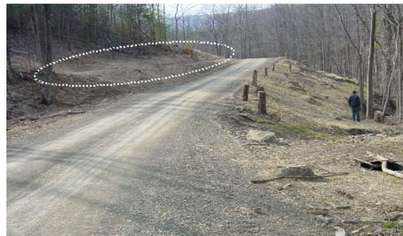
6-31 Newly constructed low-gradient bank benches.
