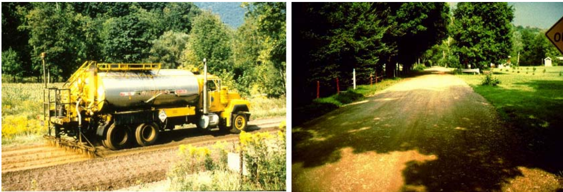
7-10 Road stabilization or full-depth reclamation works well with a stabilizing agent
