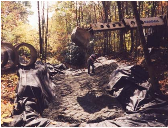
A7-04 Bedding material added
