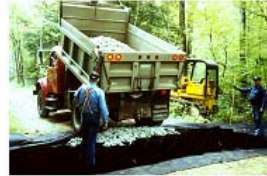
↑ Dumping aggregate fill ↑
