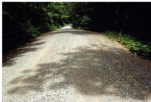
3-07A good road crown is our first line of defense against water.
