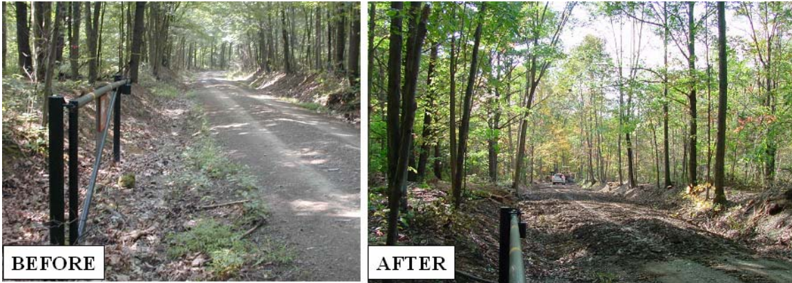
6-11 Before and after look at selective tree trimming during a road project – letting in more sunlight with less shade – striking a balance.
