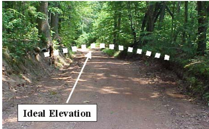
ESMP12-01 A typical entrenched road.
