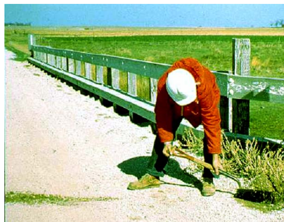
3-28 Using a shovel is the sign of a “professional operator.”
