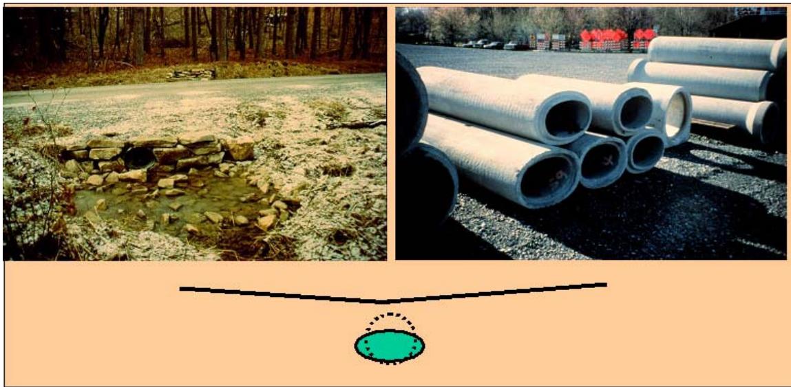
5-31 Shallow installations: use rigid pipe, squash pipe, or elliptical concrete (rigid) pipe.
