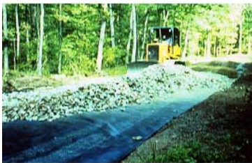
↑ Spreading the aggregate ↑
