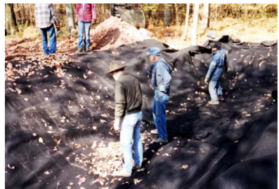
A7-03 Geotextile separation fabric laid in new trench.
