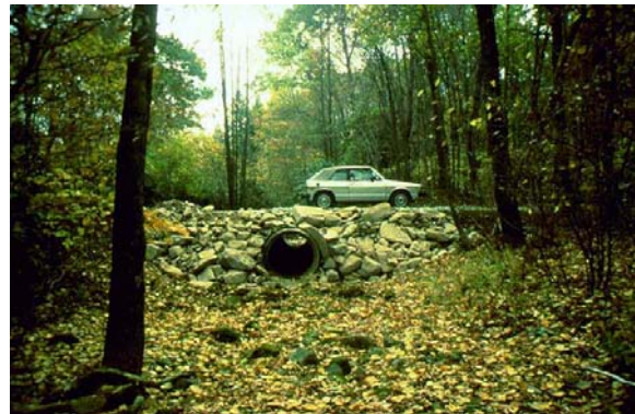
A7-09 Completed project with a leveled road stream saver system.
