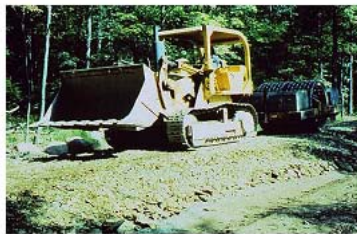
↑ Compacting the aggregate ↑
