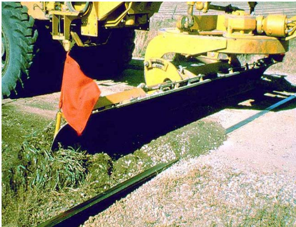
3-23 Keeping rails clean of road material is essential for safety.
