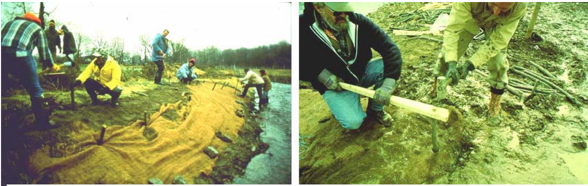
6-36 Driving the Stakes.
