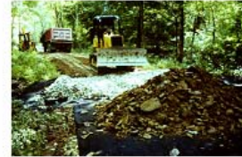
↑ Raising road elevation ↑
