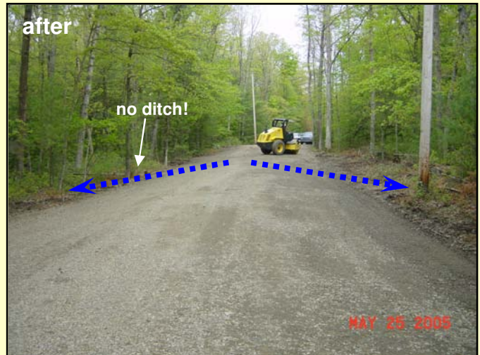
Photo 4. The road was elevated to eliminate the ditch on the left and achieve sheet flow. The added material also provided the necessary cover to install new crosspipes.
