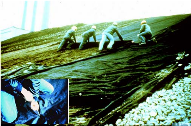
7-24 Installation of an erosion control fabric.
