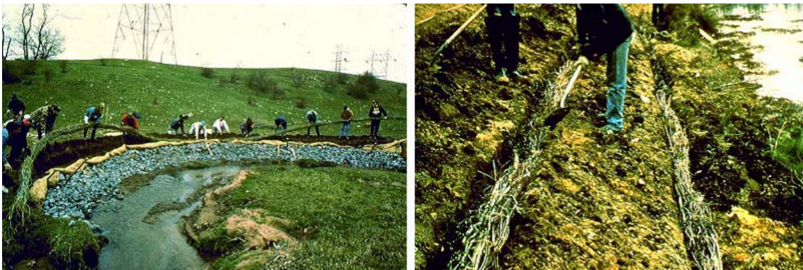
6.39 Placing the fascine and backfilling.
