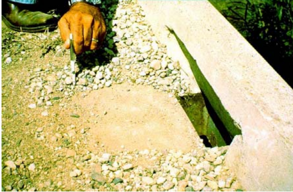
3-25 Drainage openings (scuppers) in bridge decks must be kept cleaned.
