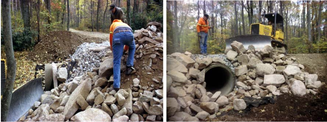
A7-08 Placing large size riprap at ends of pipe.
