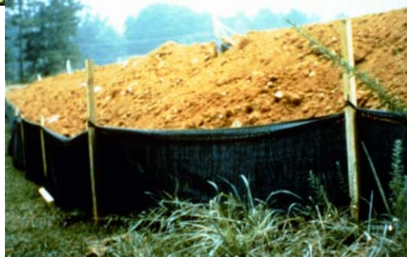
7-25 Geotextile silt fence barrier.
