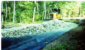
↑ Spreading the aggregate ↑
