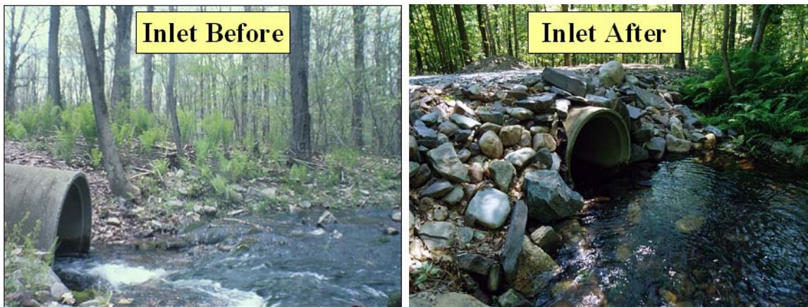
A7-10 Inlet conditions before and after project.
