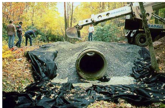
A7-07 After backfilling, fabric brought up and over pipe ends to encase entire installation.
