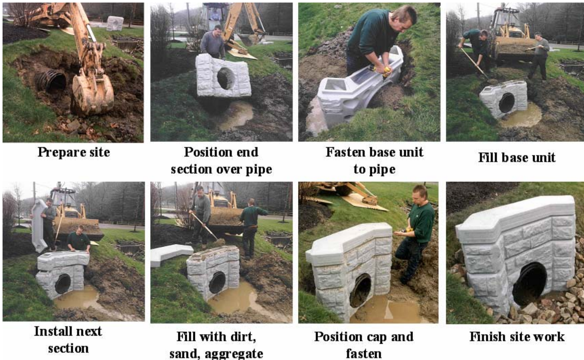
7-39 Pre-Fab Geosynthetic Endwall Installation.
