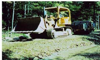
↑ Compacting the aggregate ↑
