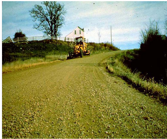
3-19 Blading or smoothing a rough surface restores rideability and prevents further more extensive deterioration.
