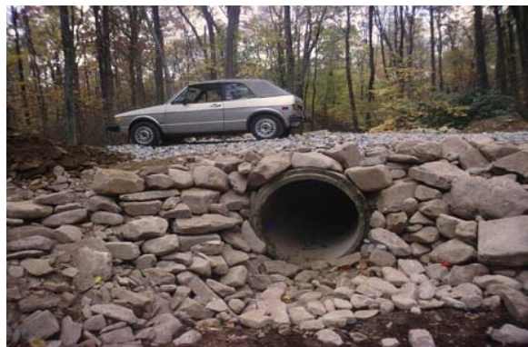
5-43 Stream Saver System – raised level road with ditch turnouts to vegetative filters.
