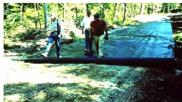
↑ Rolling out the fabric ↑
