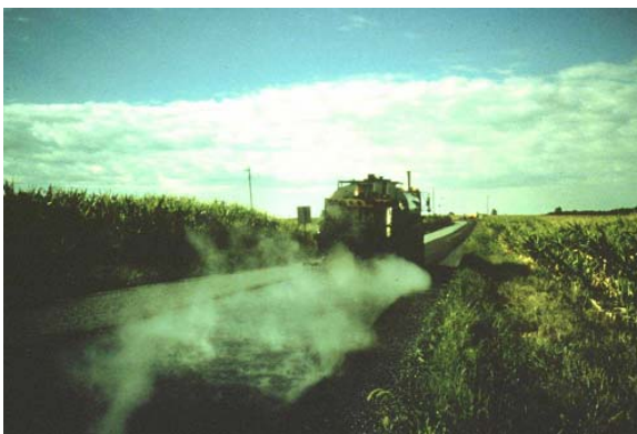
7-08 Asphalt emulsions and cutbacks are still being used for dust control, but...
