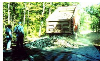
↑ Backdumping the aggregate ↑
