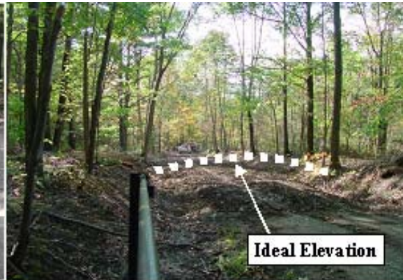
During placement of shale fill
