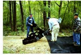
↑ Placing geocell ↑
