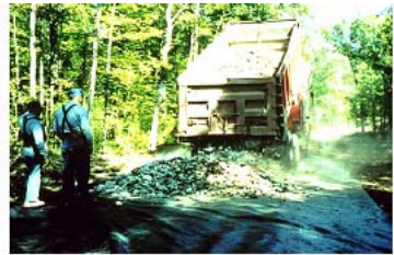
↑ Backdumping the aggregate ↑
