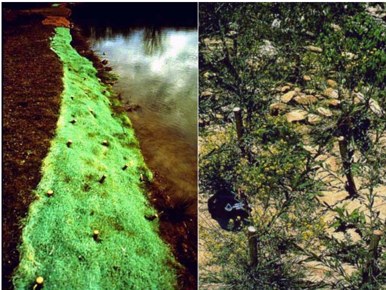
6.37 Completed site and after one season's growth.
