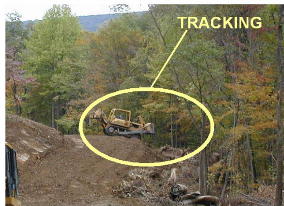
6-30 Tracking the newly constructed banks.
