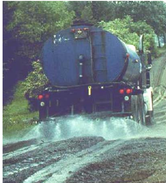
7-06 Although environmentally sensitive, water affords only short-term dust control.
