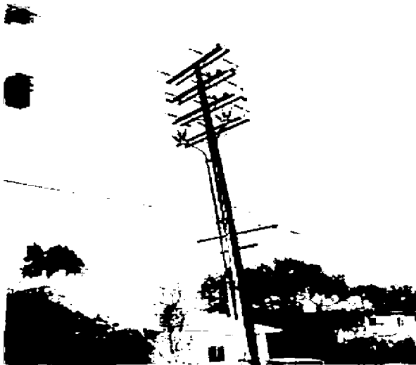
Aerial distribution lines
