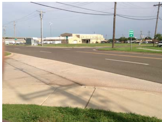
8 Accessible Route Violation 2B
