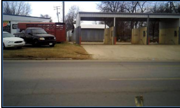
Corner 4 No Ramp (4z)
