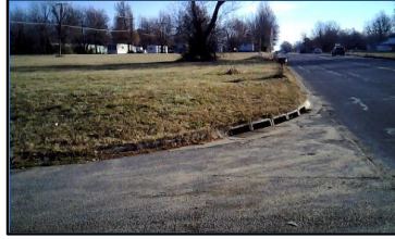
Corner 2 No Ramp (2z)
