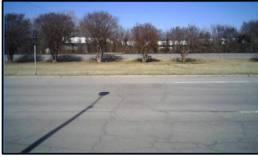
Corner 1 No Ramp (1z)
