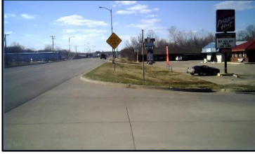
Corner 1 No Ramp (1z)
