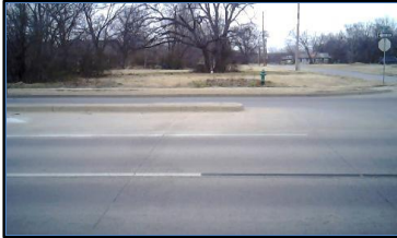
Corner 4 No Ramp (4z)
