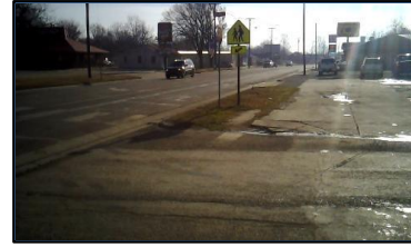
Corner 3 No Ramp (3z)
