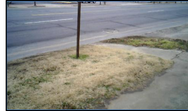
Corner 4 No Ramp (4z)
