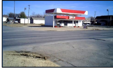
Corner 2 No Ramp (2z)
