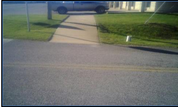
Corner 4 No Ramp (4z)
