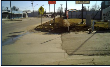
Corner 1 No Ramp (1z)
