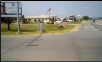
Corner 4 No Ramp (4z)
