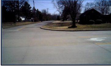
Corner 4 No Ramp (4z)
