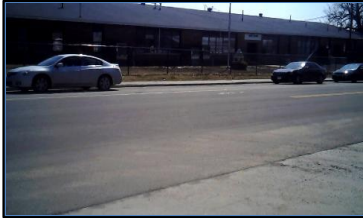
Corner 3 No Ramp (3z)
