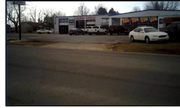
Corner 3 No Ramp (3z)
