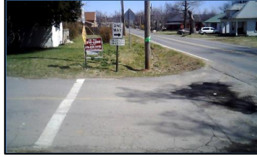
Corner 2 No Ramp (2z)
