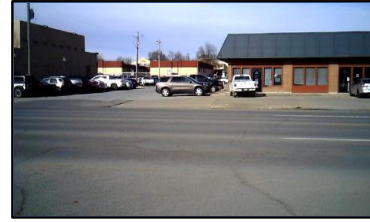
Corner 2 No Ramp (2z)
