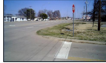
Corner 3 No Ramp (3z)
