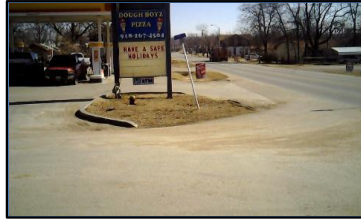
Corner 2 No Ramp (2z)
