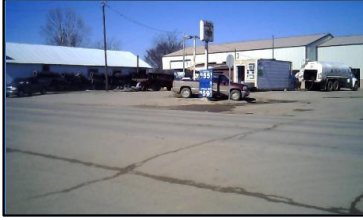
Corner 1 No Ramp (1z)
