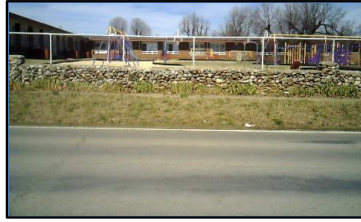
Corner 2 No Ramp (2z)
