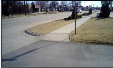
Corner 1 No Ramp (1z)
