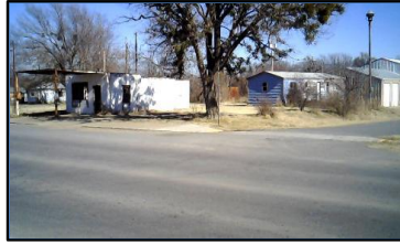
Corner 2 No Ramp (2z)
