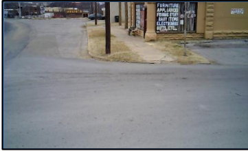
Corner 1 No Ramp (1z)
