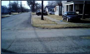
Corner 4 No Ramp (4z)
