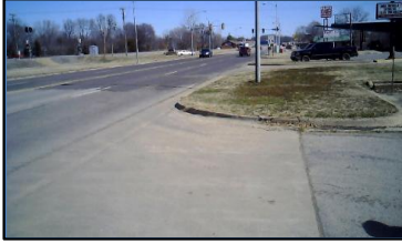
Corner 3 No Ramp (3z)
