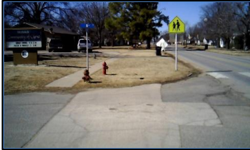
Corner 4 No Ramp (4z)
