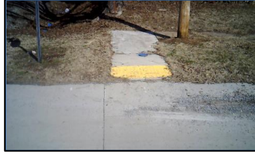
Corner 2 No Ramp (2z)
