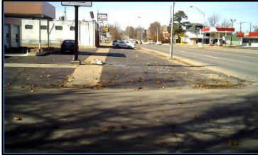
Corner 4 No Ramp (4z)
