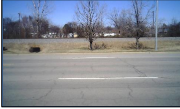
Corner 1 No Ramp (1z)
