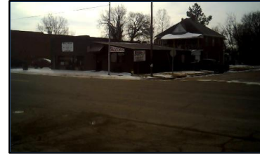
Corner 3 No Ramp (3z)
