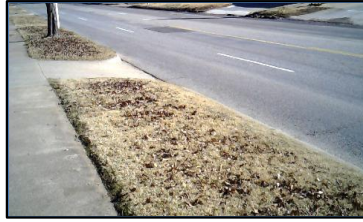
Corner 2 No Ramp (2z)
