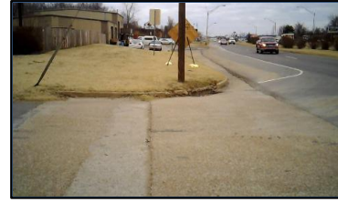
Corner 1 No Ramp (1z)
