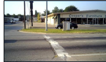
Corner 4 No Ramp (4z)
