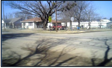
Corner 1 No Ramp (1z)
