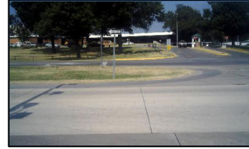
Corner 1 No Ramp (1z)
