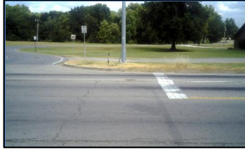
Corner 2 No Ramp (2z)
