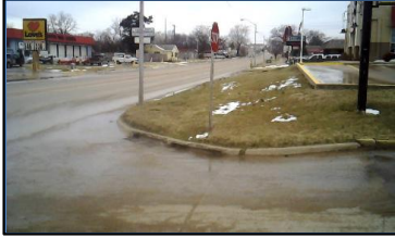
Corner 1 No Ramp (1z)
