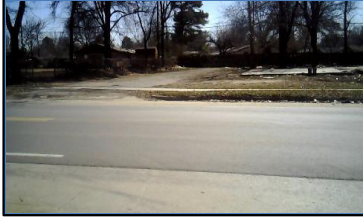
Corner 4 No Ramp (4z)
