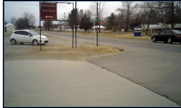
Corner 3 No Ramp (3z)
