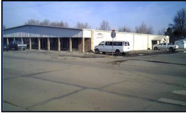
Corner 1 No Ramp (1z)
