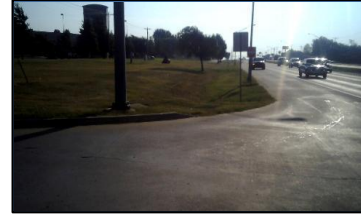
Corner 2 No Ramp (2z)
