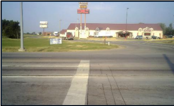
Corner 4 No Ramp (4z)
