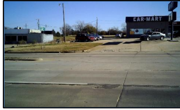
Corner 2 No Ramp (2z)
