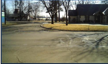
Corner 4 No Ramp (4z)
