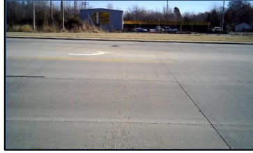
Corner 2 No Ramp (2z)
