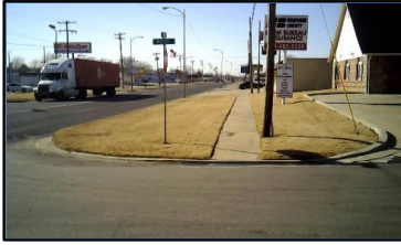
Corner 1 No Ramp (1z)
