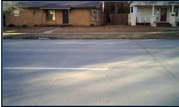
Corner 4 No Ramp (4z)
