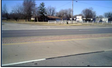
Corner 1 No Ramp (1z)
