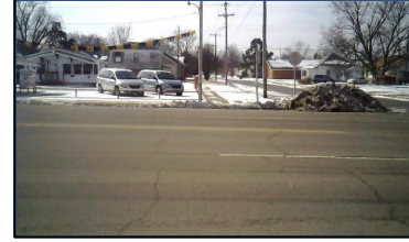
Corner 3 No Ramp (3z)
