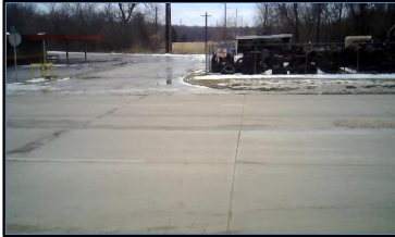
Corner 4 No Ramp (4z)
