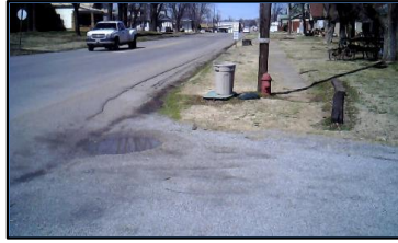
Corner 2 No Ramp (2z)
