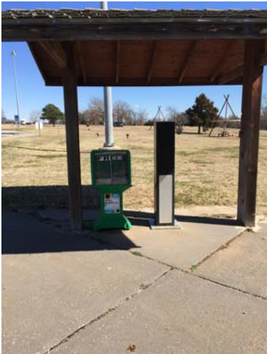
4. Accessible Route Violation 1B
