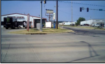
Corner 1 No Ramp (1z)
