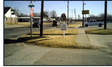
Corner 3 No Ramp (3z)
