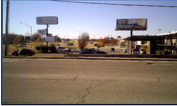
Corner 4 No Ramp (4z)
