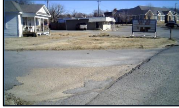
Corner 2 No Ramp (2z)
