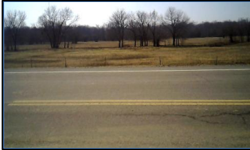
Corner 4 No Ramp (4z)
