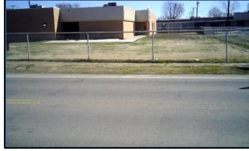
Corner 2 No Ramp (2z)
