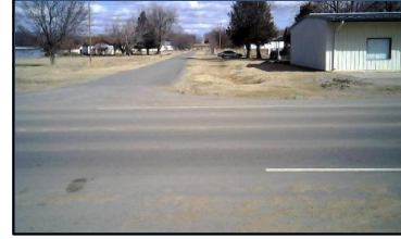
Corner 3 No Ramp (3z)
