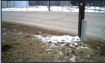
Corner 1 No Ramp (1z)
