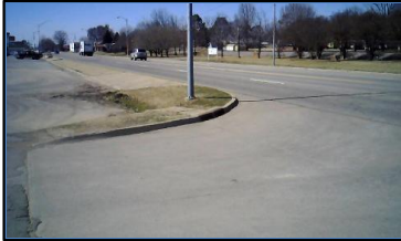
Corner 4 No Ramp (4z)
