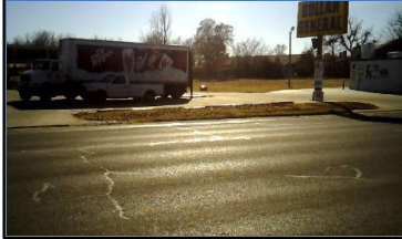
Corner 4 No Ramp (4z)
