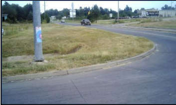
Corner 2 No Ramp (2z)
