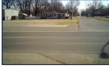
Corner 2 No Ramp (2z)
