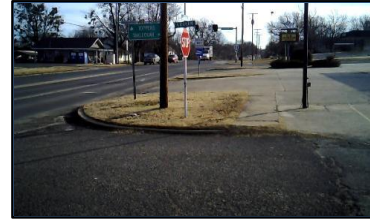
Corner 3 No Ramp (3z)
