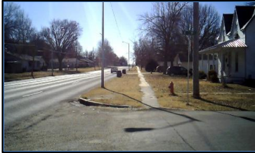
Corner 4 No Ramp (4z)
