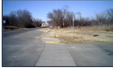
Corner 2 No Ramp (2z)
