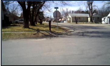
Corner 4 No Ramp (4z)
