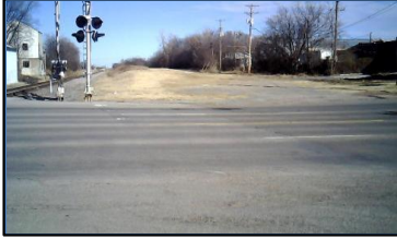
Corner 1 No Ramp (1z)
