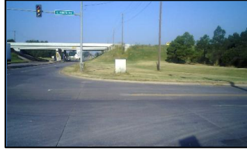
Corner 1 No Ramp (1z)
