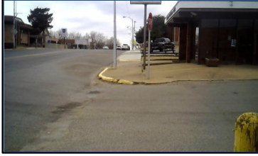
Corner 1 No Ramp (1z)
