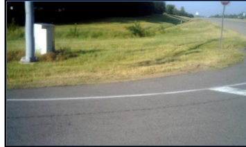
Corner 4 No Ramp (4z)
