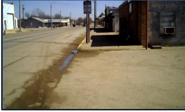
Corner 3 No Ramp (3z)
