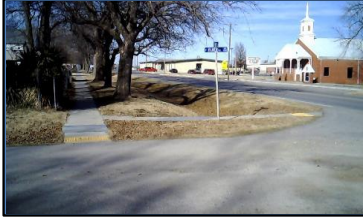
Corner 1 No Ramp (1z)
