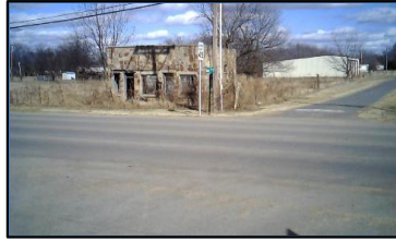
Corner 2 No Ramp (2z)
