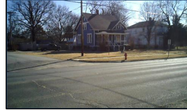
Corner 3 No Ramp (3z)
