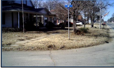
Corner 4 No Ramp (4z)
