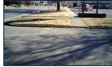
Corner 3 No Ramp (3z)
