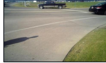
Corner 3 No Ramp (3z)
