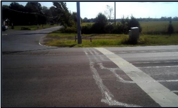
Corner 3 No Ramp (3z)
