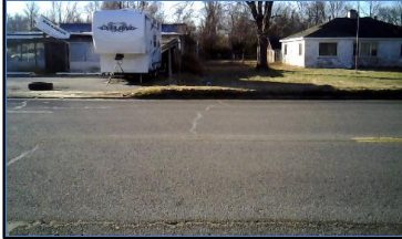
Corner 4 No Ramp (4z)
