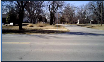
Corner 4 No Ramp (4z)
