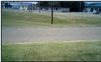
Corner 4 No Ramp (4z)
