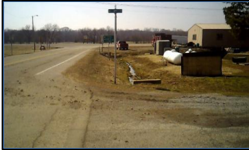
Corner 4 No Ramp (4z)
