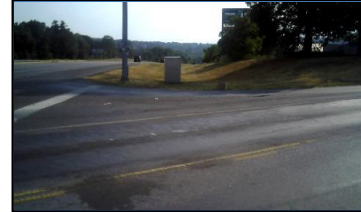
Corner 4 No Ramp (4z)
