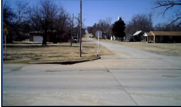
Corner 4 No Ramp (4z)
