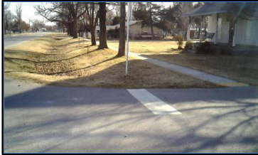
Corner 4 No Ramp (4z)
