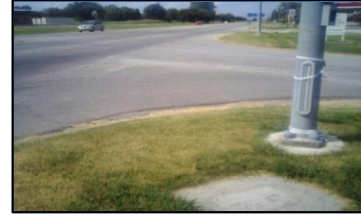
Corner 3 No Ramp (3z)
