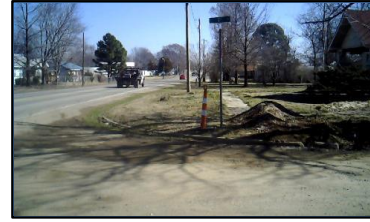
Corner 3 No Ramp (3z)
