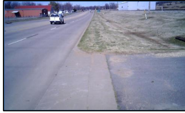
Corner 2 No Ramp (2z)
