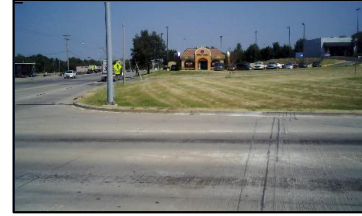
Corner 2 No Ramp (2z)
