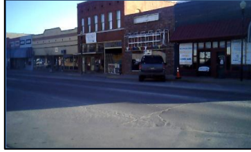
Corner 2 No Ramp (2z)
