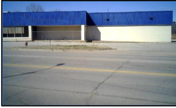
Corner 1 No Ramp (1z)
