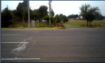
Corner 4 No Ramp (4z)
