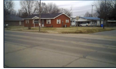
Corner 3 No Ramp (3z)
