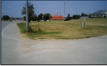
Corner 1 No Ramp (1z)
