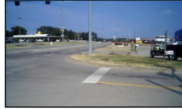
Corner 3 No Ramp (3z)
