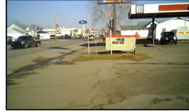
Corner 3 No Ramp (3z)
