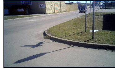
Corner 3 No Ramp (3z)
