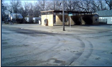
Corner 4 No Ramp (4z)
