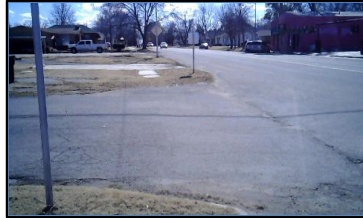
Corner 3 No Ramp (3z)
