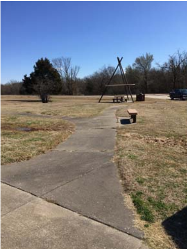
5. Accessible Route Violation 1C
