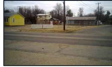
Corner 3 No Ramp (3z)
