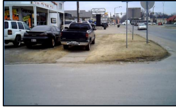
Corner 2 No Ramp (2z)
