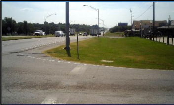
Corner 4 No Ramp (4z)
