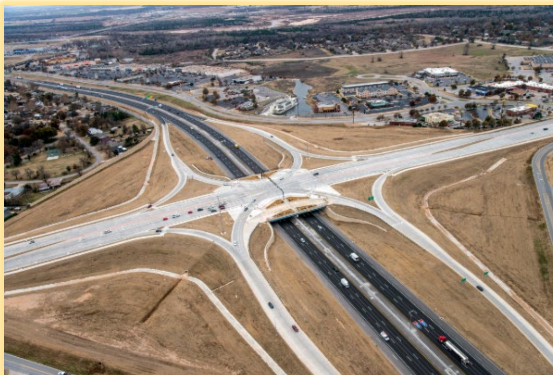
Figure 12: ODOT's recently completed SPUI interchange at I-35 & Main Street in Norman, OK
