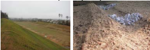
Includes: cut/fill slopes, drainage ditches, sediment basins, road beds ...
