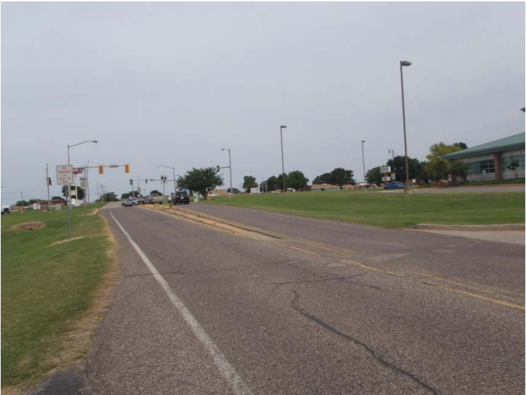
Photograph 9: Facing east along SH-74 near eastern end of study area.
