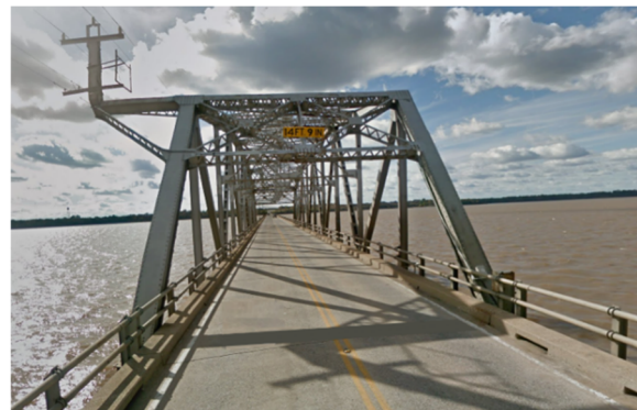
Figure 2: Truss Structure on Bridge
