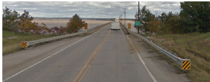
West Terminus of Bridge
