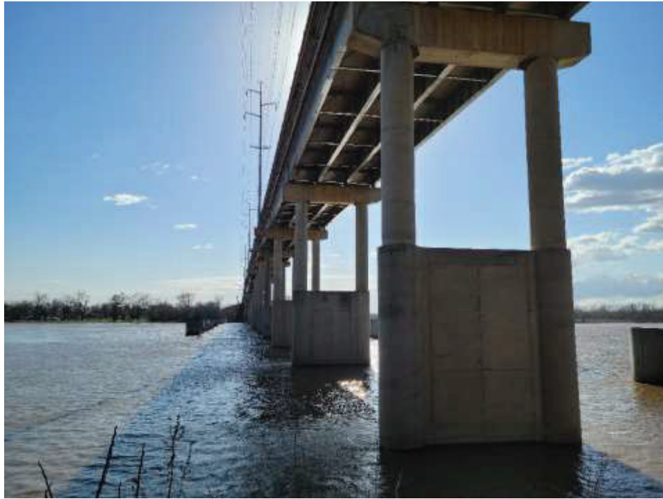
Photograph 7: A southwest-facing view of the Arkansas River and SH-100 bridge.
