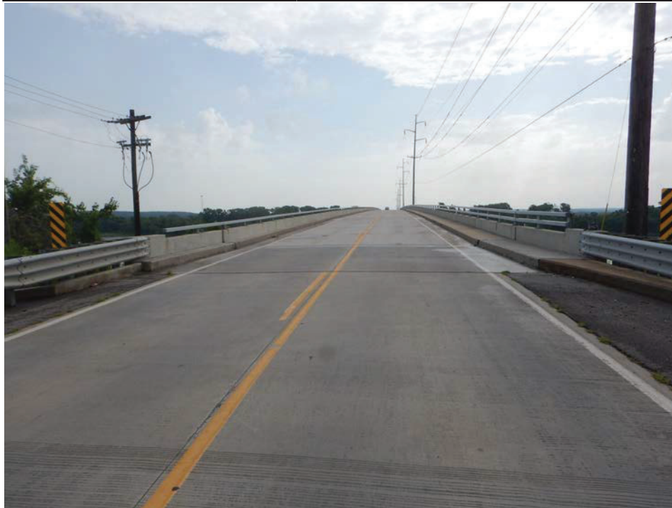
Photograph 1 - Looking east at the bridge end view.
