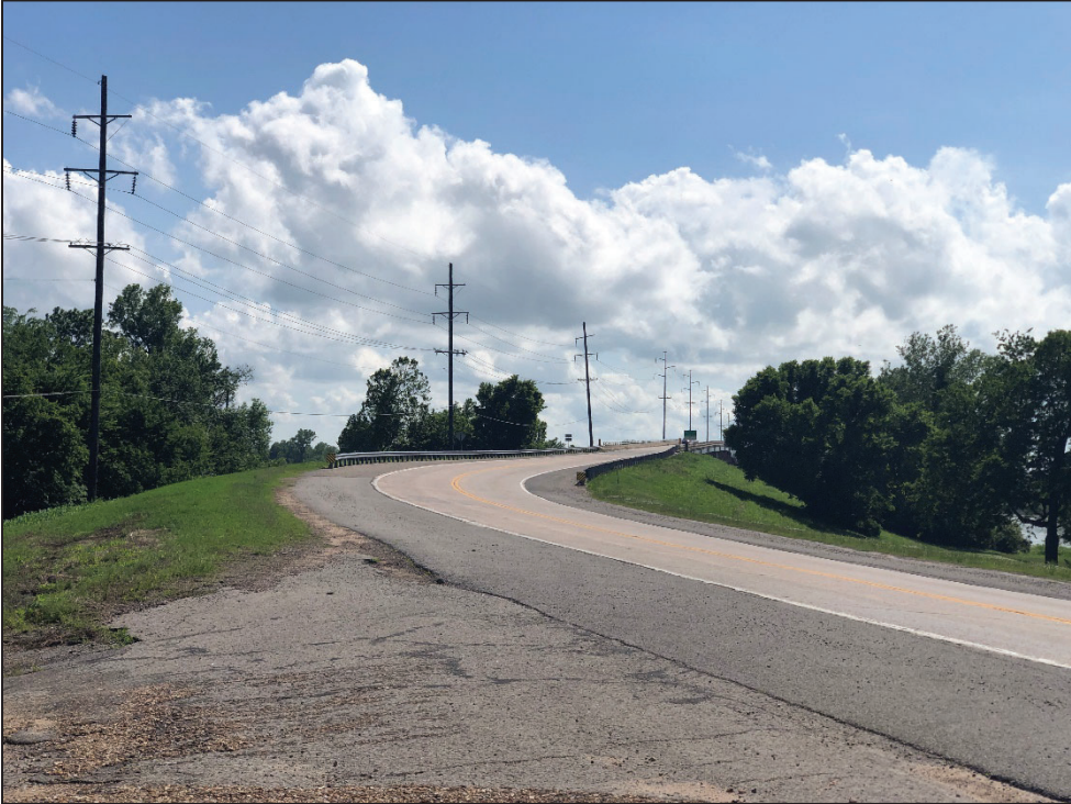
Photo 1: Looking southwest at the SH-100 bridge from the northern project terminus in Gore.
