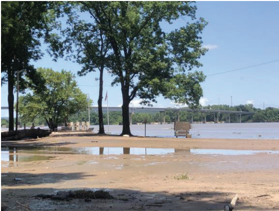
1. View looking north at the Arkansas River Bridge. Photograph taken from the east side of SH-100 in the flooded Webbers Falls City Park.
