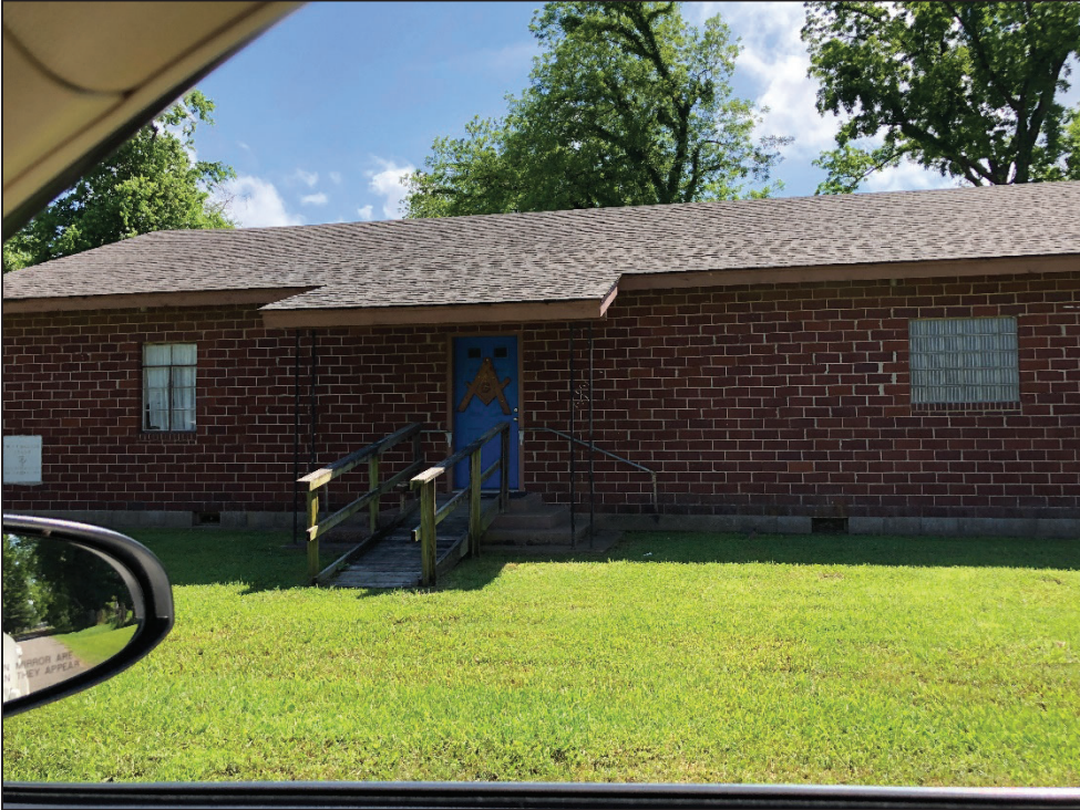
Photo 15: Webbers Falls Mason Lodge on N Main Street in Webbers Falls.
