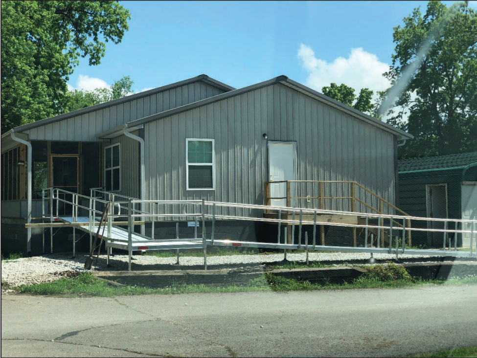
Photo 13: Home with ramp in the study area.
