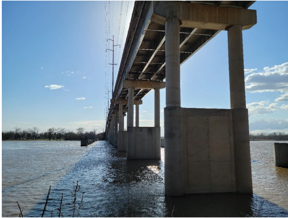
Photograph 9: A southwest-facing view of the Arkansas River and SH-100 bridge.
