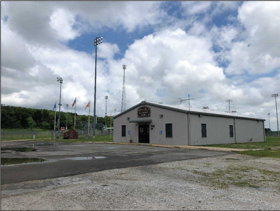
Photo 30: Gore Community and Senior Citizen's Center located on Steve Owens Road.
