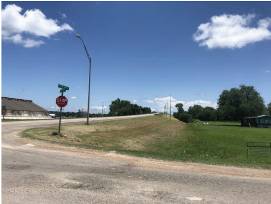
15. View looking northwest at the northeast bound side of SH-100. Photograph taken from the south side of SH-100 at Standwaite Blvd.
