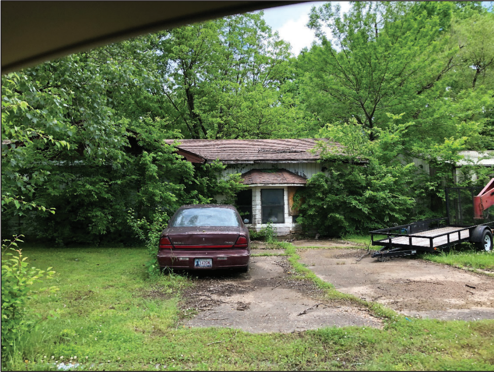
Photo 33: Home in disrepair in the study area.
