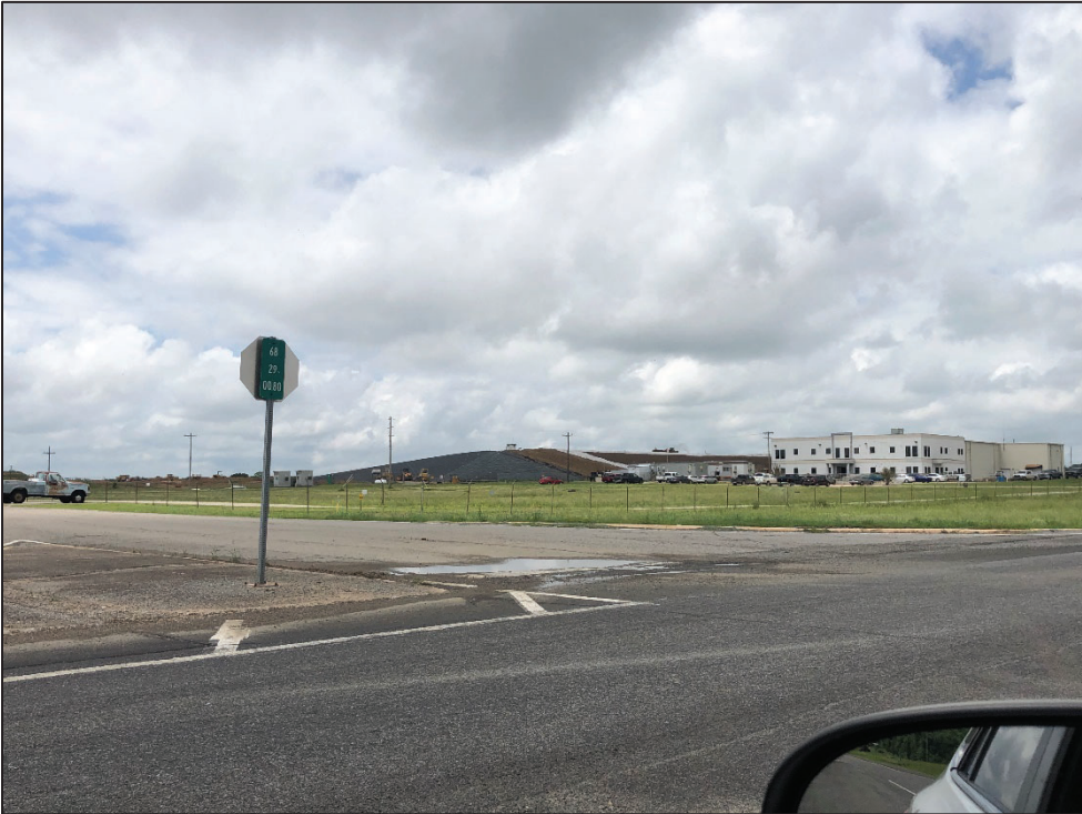
Photo 28: Electric substation on the west side of SH-10.
