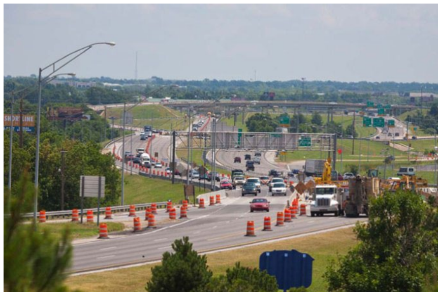
FIGURE 7: SMART WORK ZONE EXAMPLE: I-244 IN TULSA, OKLAHOMA
