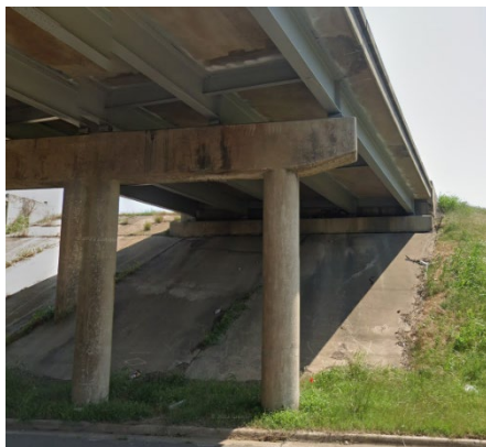
Existing pier conditions - 2022
