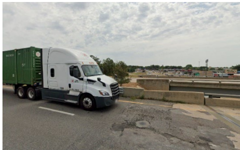
Existing deck conditions - 2022
