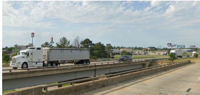
US-69 Bridge over Main Street in Durant, Oklahoma
