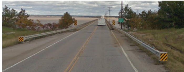
West Terminus of Bridge
