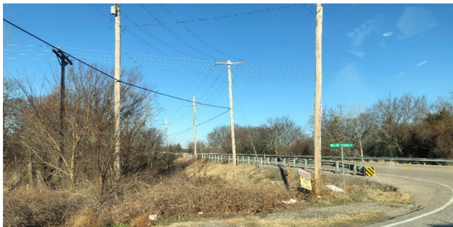
Visibility, looking West – from Stop Bar at Willow Springs Rd.
