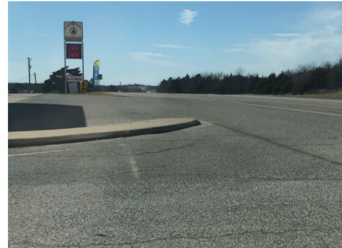
Figure 4: Visibility, looking West – from Stop Bar at State Park Road
