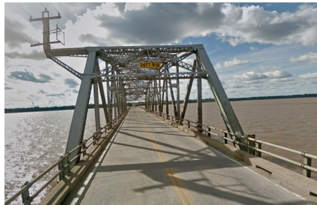
Truss Structure on Bridge
