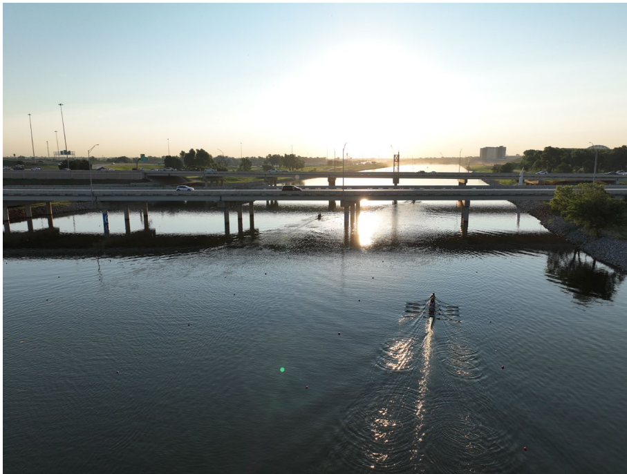
Figure 4: Rowers approaching the existing bridge pier obstructions
