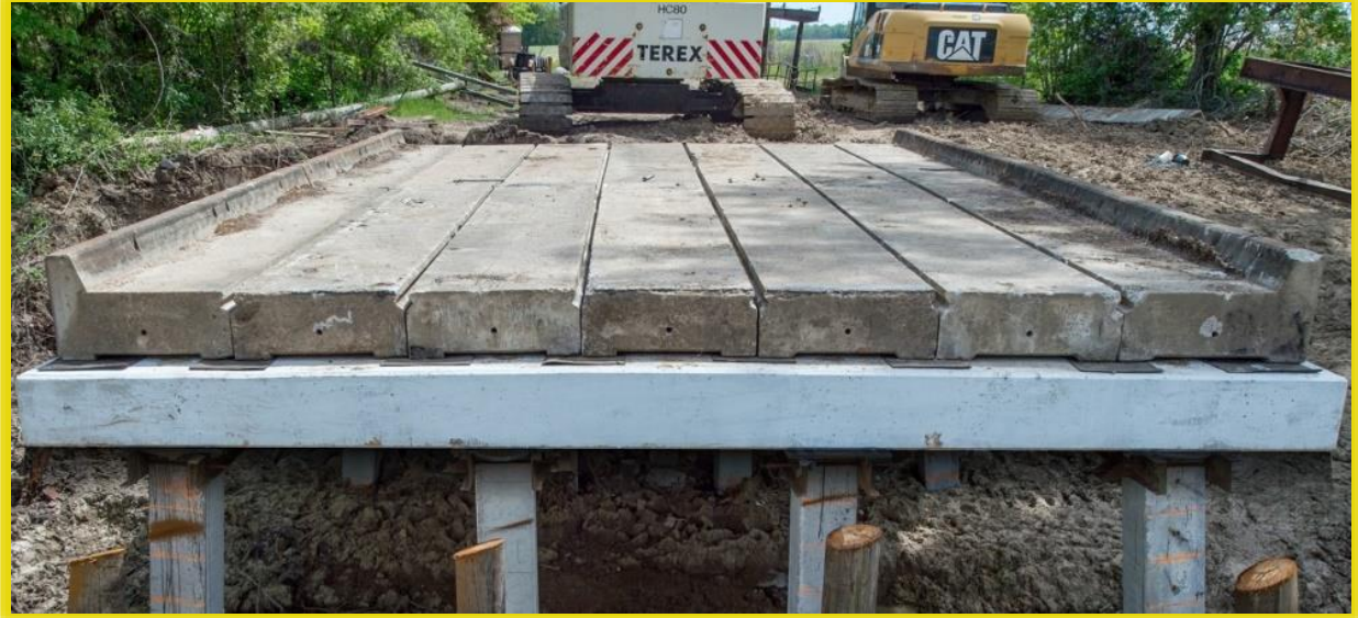
Figure 15 – Bridge with pre-cast components, Mississippi
