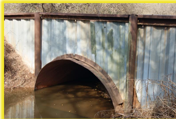
Figure 5: Temporary Arch Pipe Bridge
