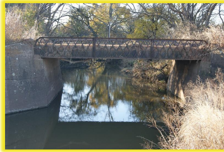
Figure 3: Existing I-Beam Span Bridge
