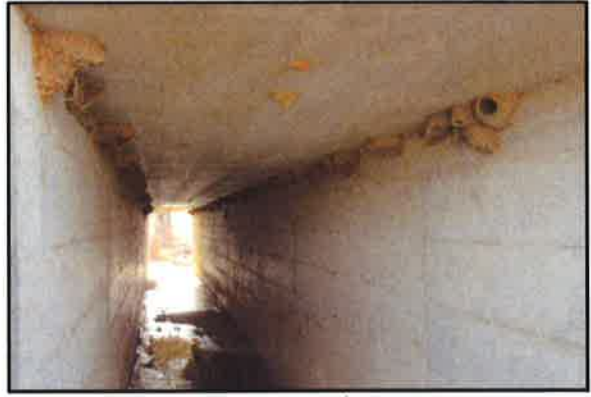
Photograph 8: Swallow Nests in Culvert
