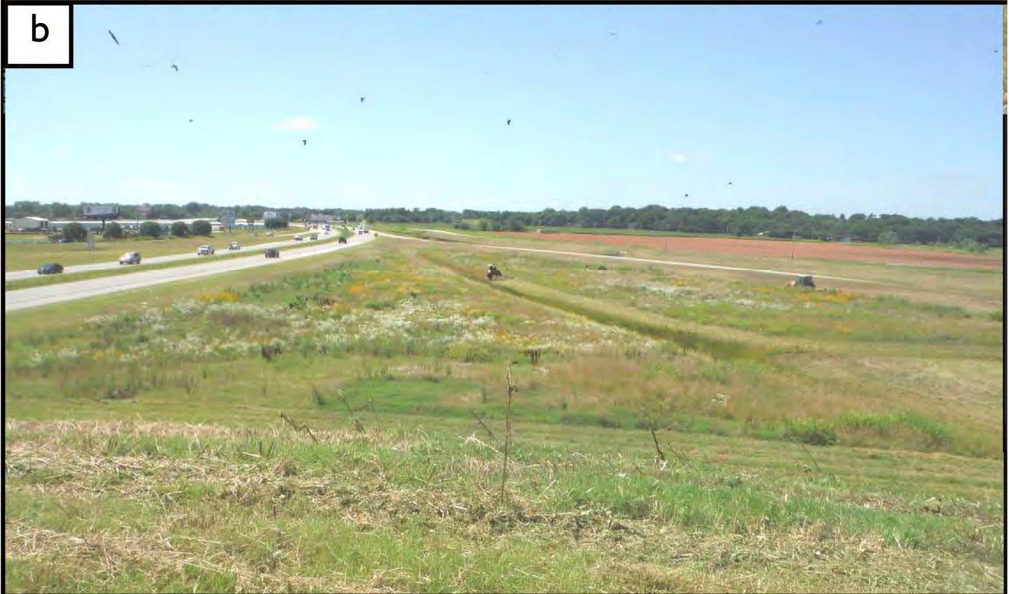
Figure 6. Disturbed ROW at I-35/SH-9 intersection between the highway and ramps in the area of the former cloverleaf, view northwest (a); and view southeast (b).
