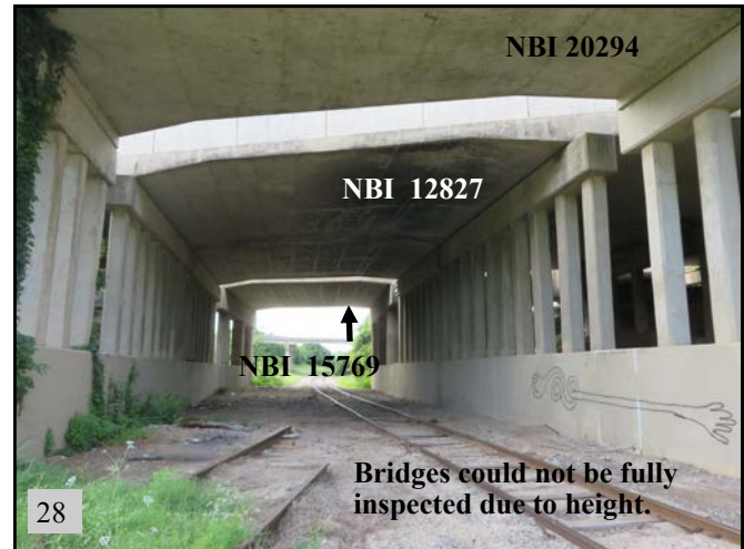
▲ (PS 17): View of NBIs 20294, 12827, and 15769. View is to the southeast.
