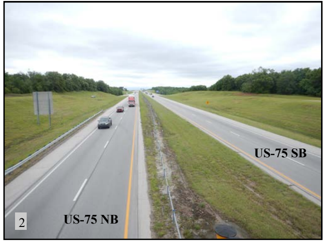
▲ (PS 2): View of US-75 from the W. 61st Street bridge (NBI 16564). View is to the south.
