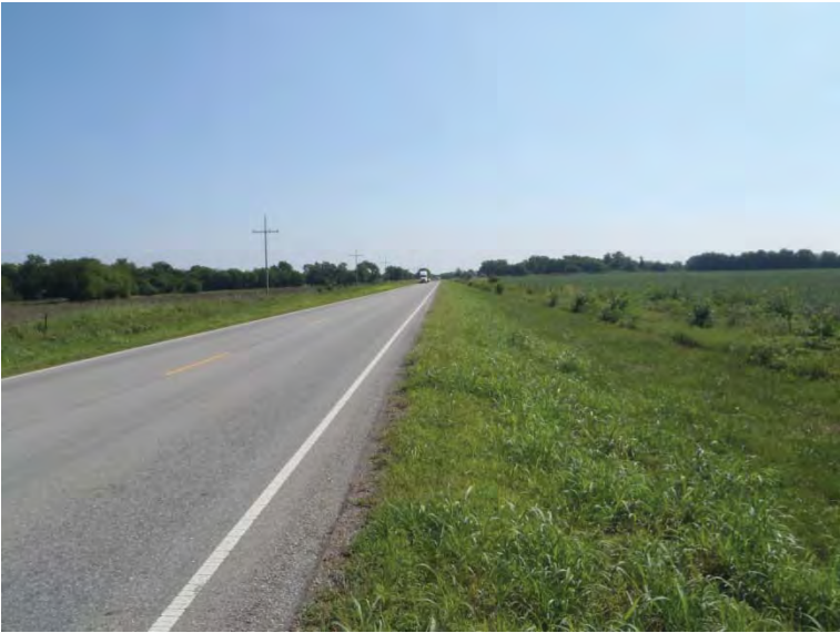
Photograph 31: Facing northeast along SH-48 near northern edge of study area.
