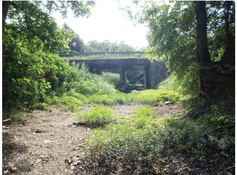
Photograph 8: Facing east from within FS-4.
