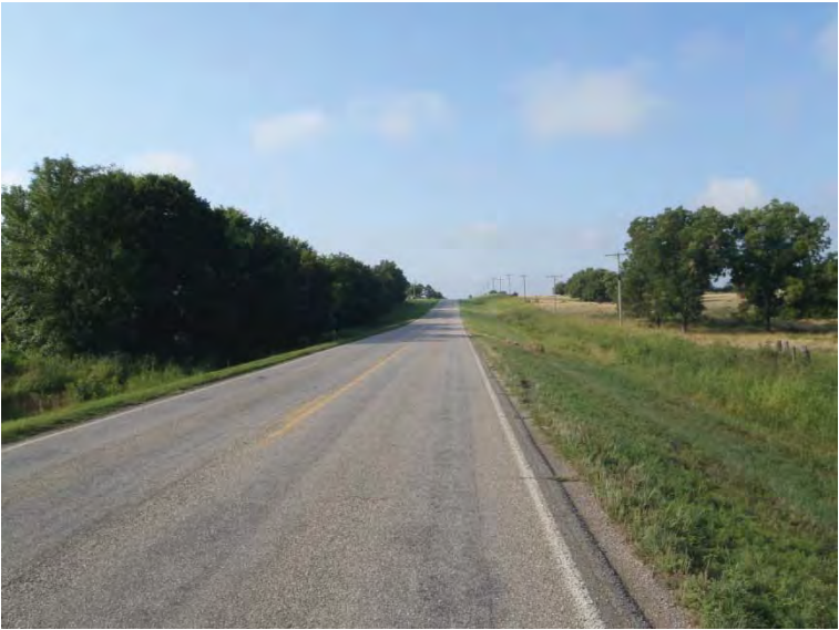
Photograph 1: Facing south along SH-48 near southern edge of study area.
