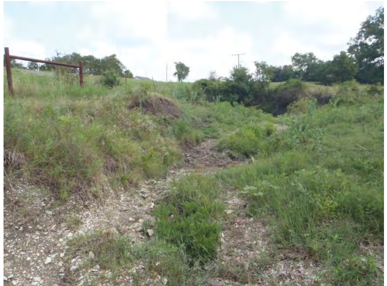
Photograph 14: Facing north from within FS-9.
