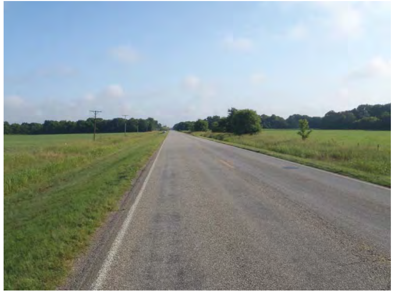
Photograph 2: Facing north along SH-48 near southern edge of study area.
