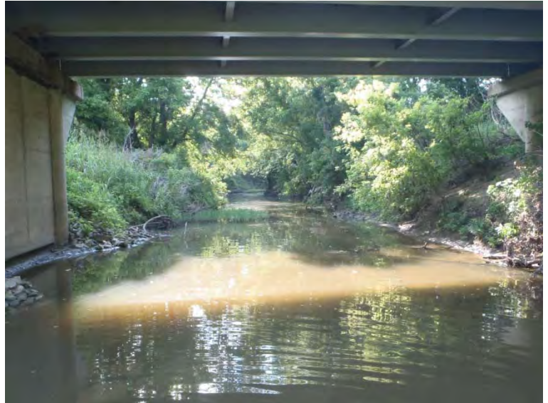
Photograph 4: Facing east from within FS-1.
