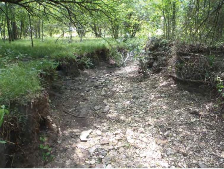
Photograph 21: Facing east from within FS-14.
