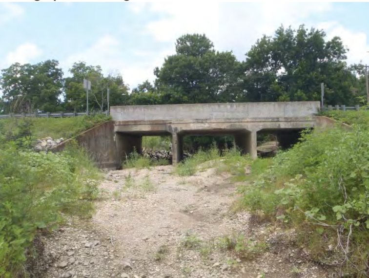
Photograph 23: Facing west from within FS-15.
