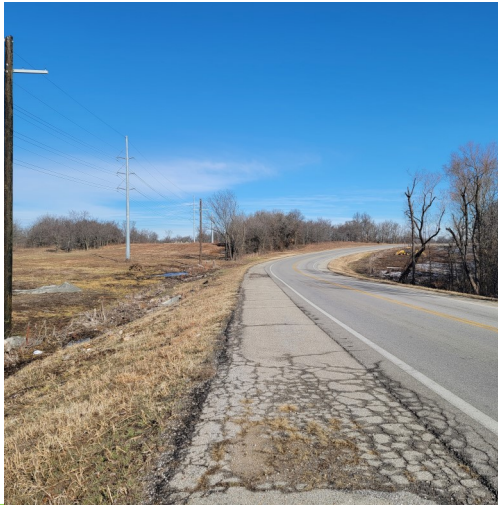
13. Point 4 looking north.
