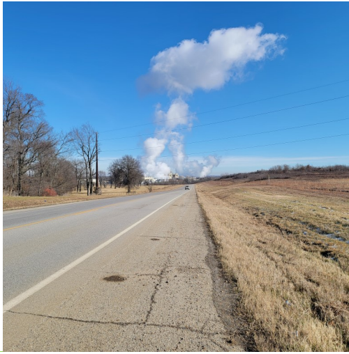
1. Point 1 looking north down SH-412B.
