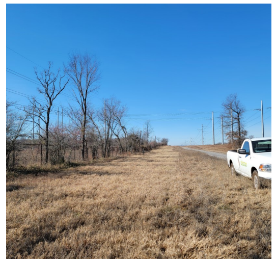
24. Point 6 looking to west.
