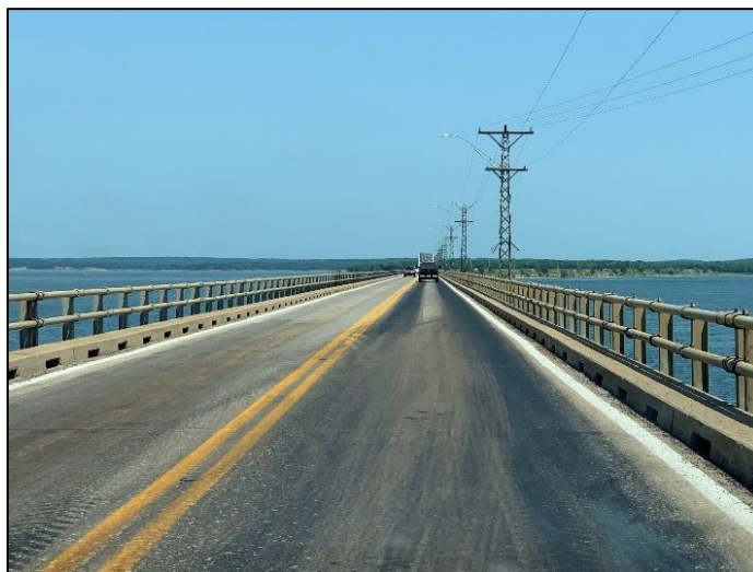
Figure 11: Narrow Deck on Roosevelt Bridge
