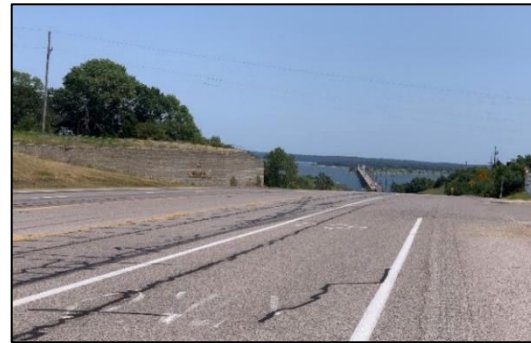
Figure 7: Roadway Intersection at State Park Rd.
