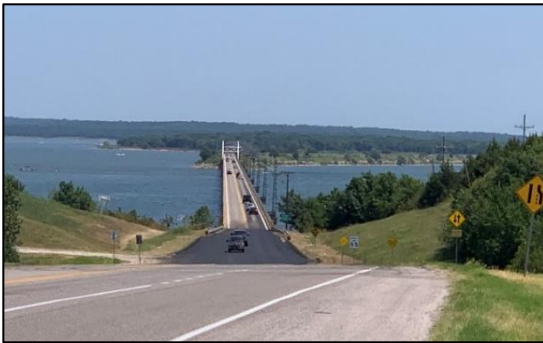
Figure 6: Western Approach Roadway Grade (Looking East)
