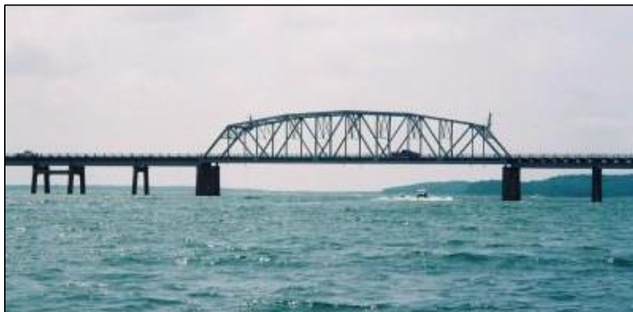
Figure 15: Roosevelt Bridge Truss Span
