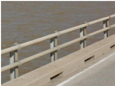
Figure 53: Existing Metal Bridge Rail
