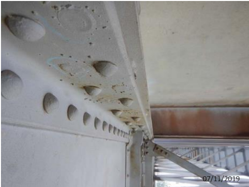
Figure 24: Inspection Photo: Primary Girder Plug Welds
