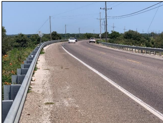
Figure 12: Horizontal Curve on Causeway (Looking East)
