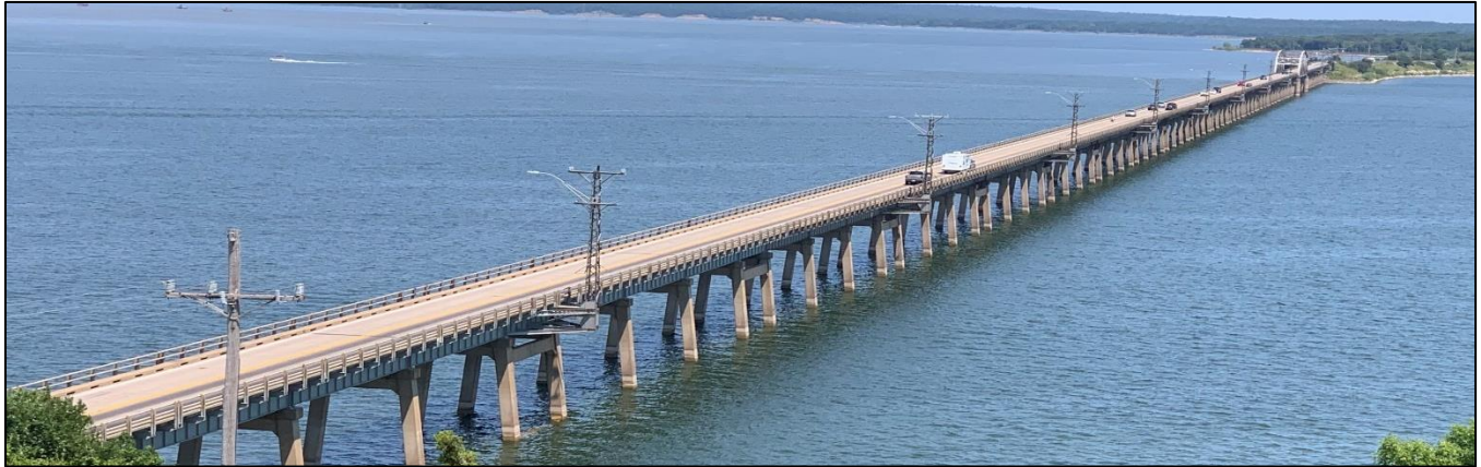
Figure 8: Segment 2 - Roosevelt Bridge (Looking East)
