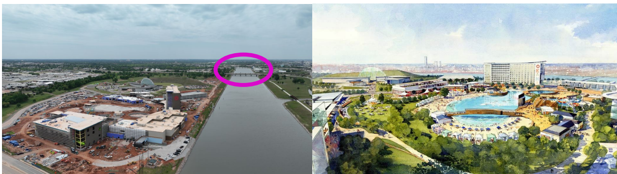
Figure 2. OKANA Resort Site Construction as of April 2024 and Rendering
