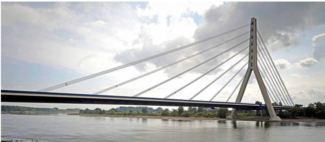
FIGURE 12 – CABLE-STAYED BRIDGE (FLEHE BRIDGE)
