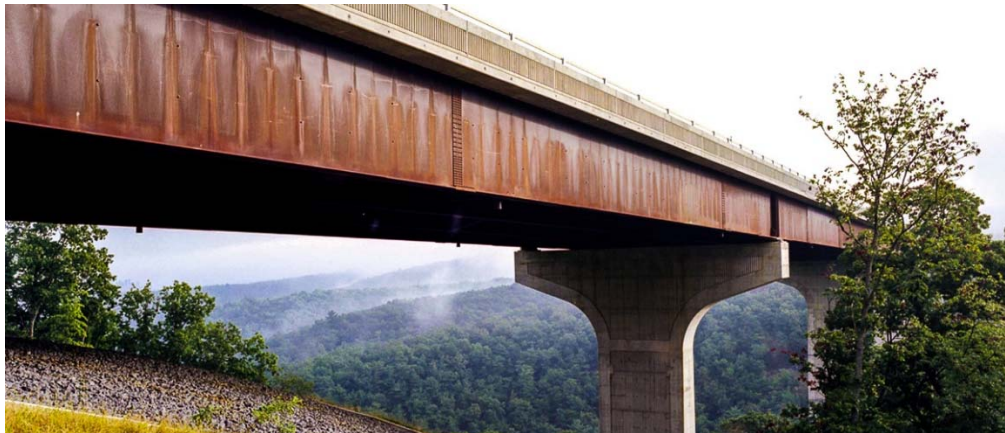
FIGURE 7 – STEEL PLATE GIRDER BRIDGE
