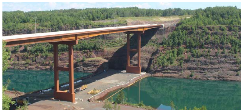
Figure 2.2: Rouchleau Mine Bridge, Eveleth, MN
