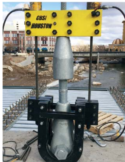
FIGURE 16 – ADJUSTABLE SINGLE STRAND HANGER INSTALLATION
