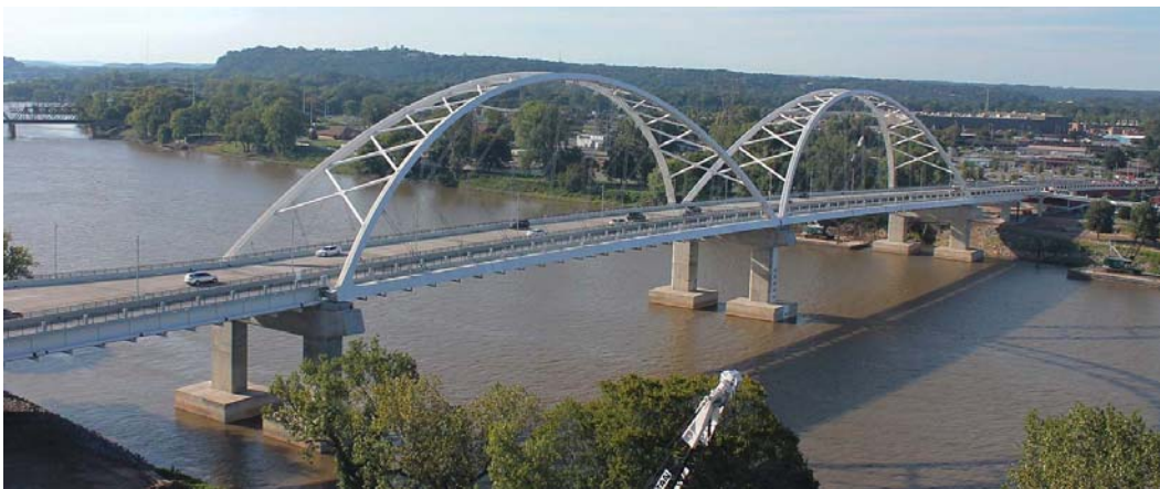
FIGURE 11 – TIED ARCH BRIDGE (BROADWAY BRIDGE)
