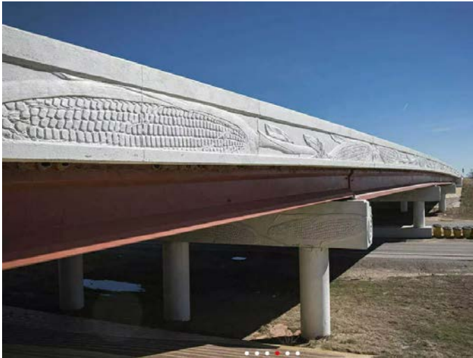
Figure 8.1: SH-9 Bridge, Norman, OK
