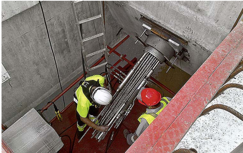
FIGURE 26 – CABLE STAY INSTALLATION
