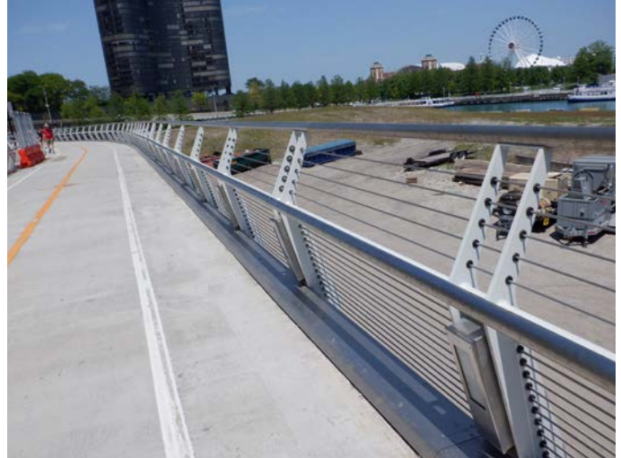
Figure 5.5: Lakefront Trail Bridge, Chicago, IL
