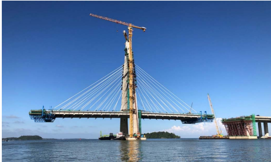
FIGURE 27 – CABLE-STAYED BRIDGE CONSTRUCTION (TEMBURONG BRIDGE)
