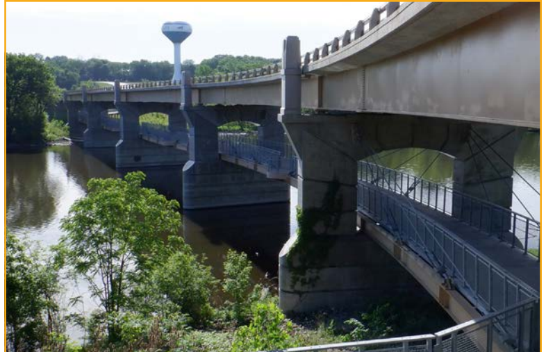
Figure 1.3: Red Gate Road over the Fox River, St. Charles, IL
