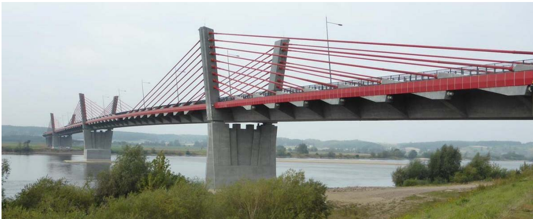
FIGURE 9 – EXTRADOSED BRIDGE (KWIDZYN BRIDGE)
