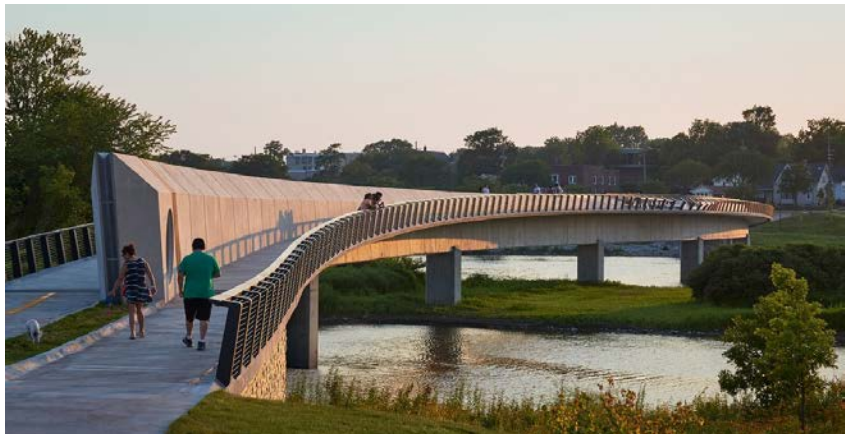
Figure 3.2: RiverEdge Bridge, Aurora, IL
