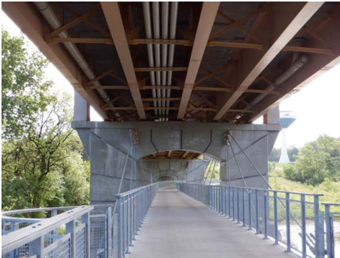
Figure 8.3: Red Gate Road over the Fox River, St. Charles, IL
