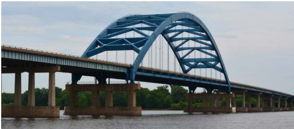
FIGURE 15 – BRIDGE WITH VERTICAL ARCH RIBS (I-280)
