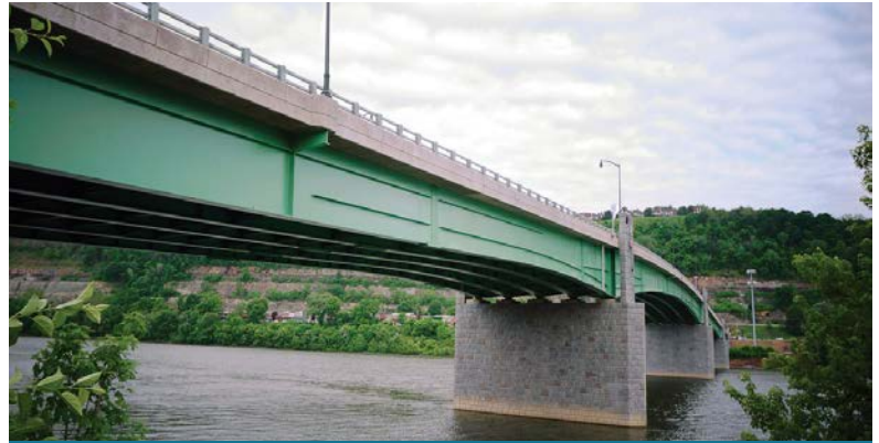
Figure 2.1: Hulton Bridge Over the Allegheny River, Allegheny County, PA
