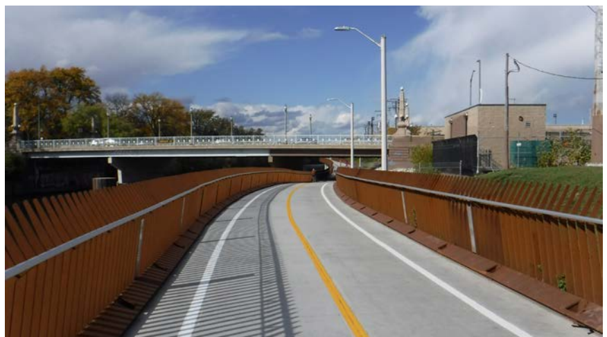
Figure 9.3: Addison Pedestrian Bridge, Chicago, IL
