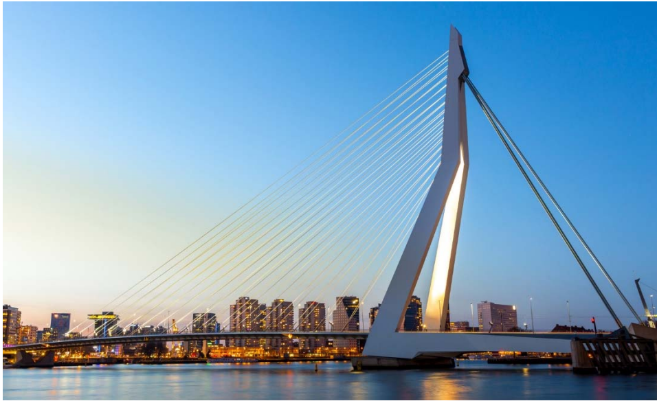
FIGURE 23 – CABLE-STAYED BRIDGE WITH ANGLED TOWER (ERASMUS BRIDGE)
