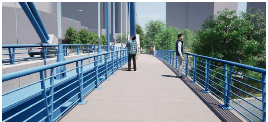
Figure 9.2: Throop Street Bridge, Chicago, IL
