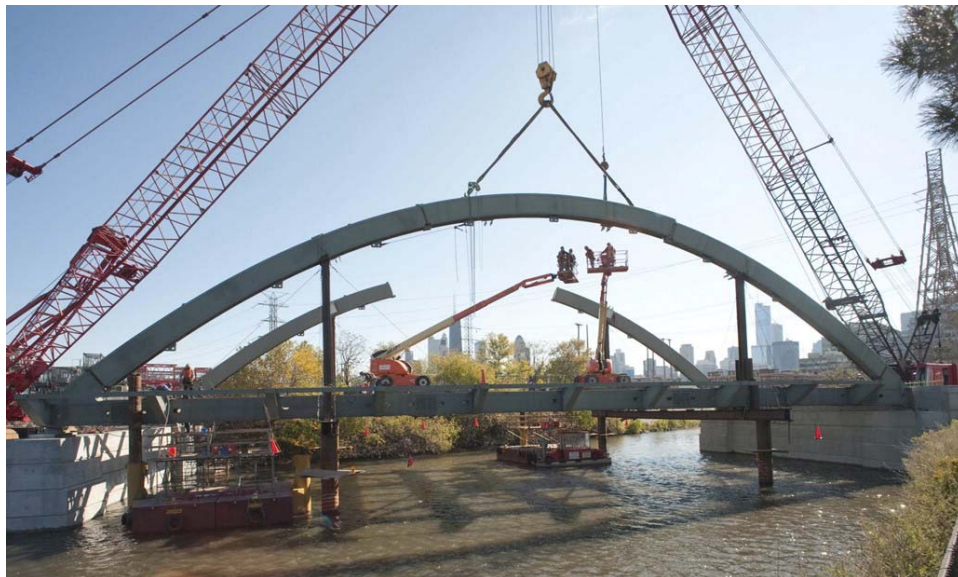
FIGURE 17 – ARCH ERECTION ON FALSEWORK (HALSTED BRIDGE)
