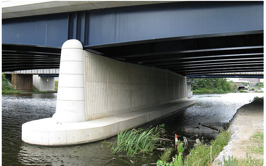
Figure 1.1: Surtees Bridge, Stockton-On-Tees, United Kingdom
