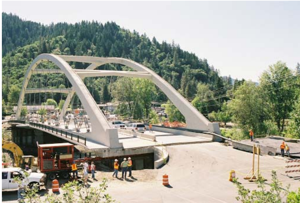
FIGURE 20 – LATERAL ROLL IN ARCH PLACEMENT (DEPOT STREET BRIDGE)
