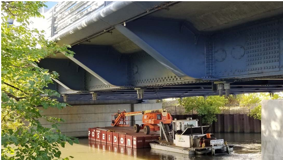
FIGURE 21 – INSPECTION EQUIPMENT FOR UNDERSIDE OF TIED ARCH (HALSTED BRIDGE)
