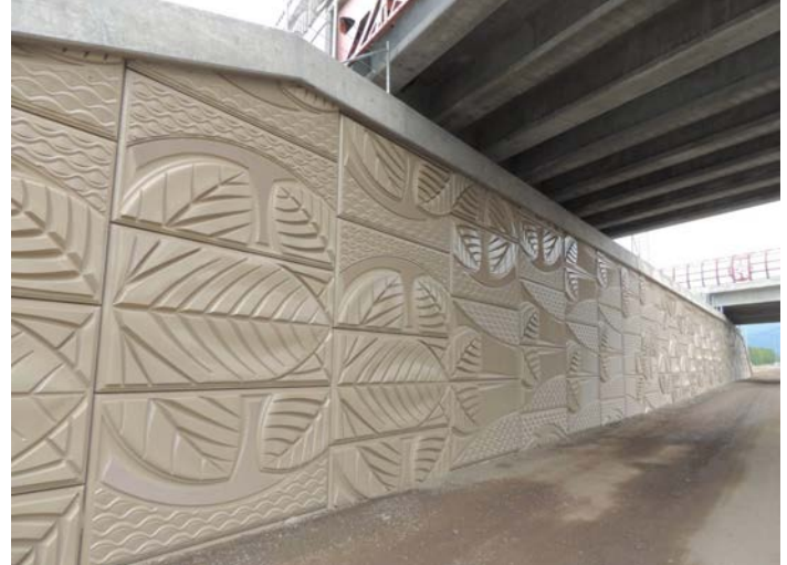
Figure 8.5: Glenn Highway and Muldoon Road, Anchorage, AK
