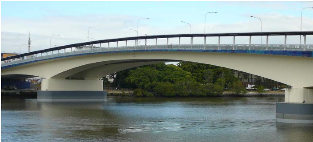
FIGURE 8 – SEGMENTAL CONCRETE BRIDGE (GO BETWEEN BRIDGE)
