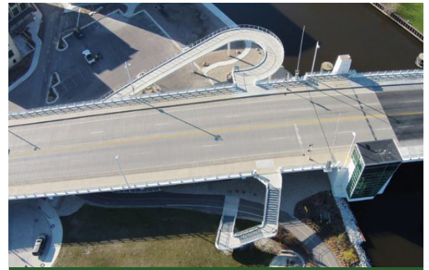
Figure 11.2: Menomonee Valley Bike Path Bridge, Milwaukee, WI
