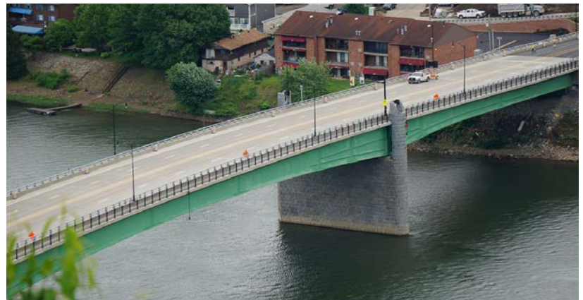
Figure 9.5: Hulton Bridge Over the Allegheny River, Allegheny County, PA
