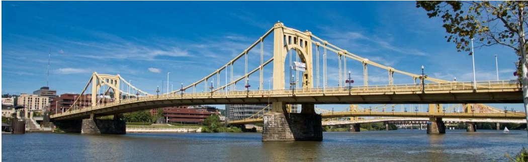
FIGURE 13 – SUSPENSION BRIDGE (ROBERTO CLEMENTE BRIDGE)
