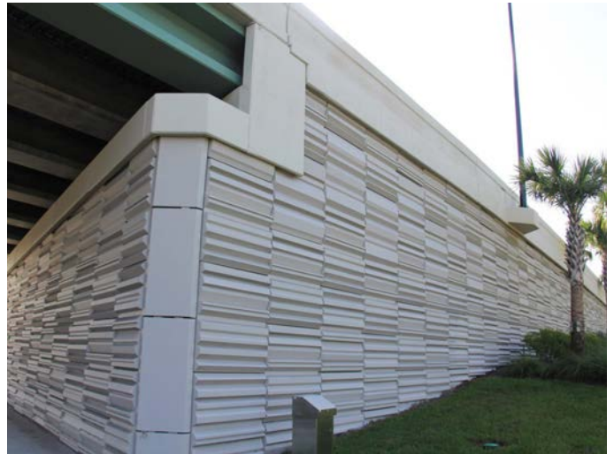
Figure 8.4: Epcot Center Drive, Orlando, FL
