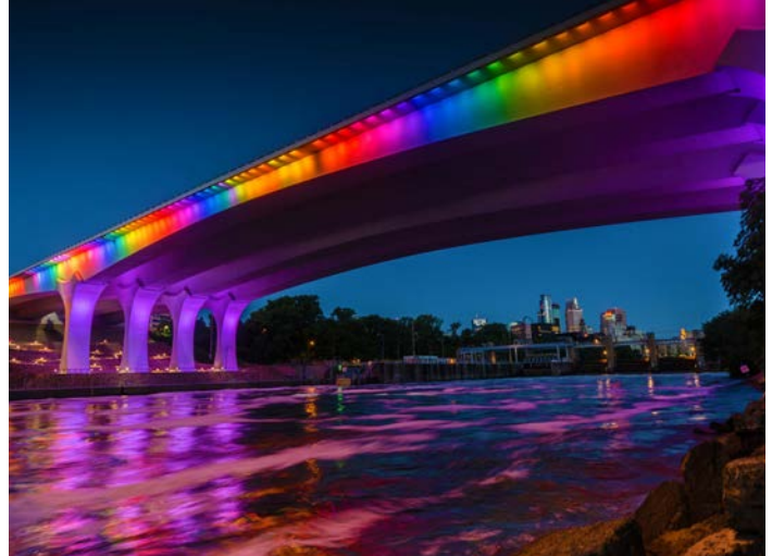
Figure 6.5: I35 W. Bridge, Minneapolis, MN
