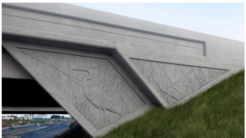
Figure 10.3: I-5/French Camp Road Bridge, Sockton, CA
