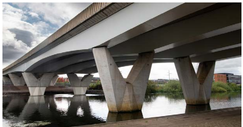
Figure 2.3: Nene Bridge, Peterborough, United Kingdom
