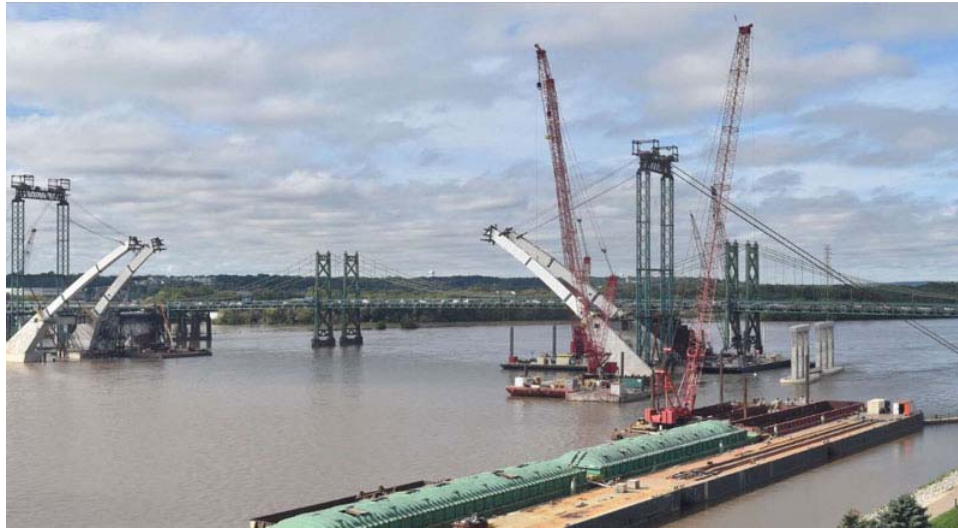
FIGURE 18 – ARCH ERECTION WITH BACK STAYS (I-74)
