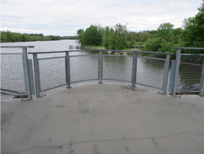
Figure 4.1: Red Gate Road over the Fox River, St. Charles, IL
