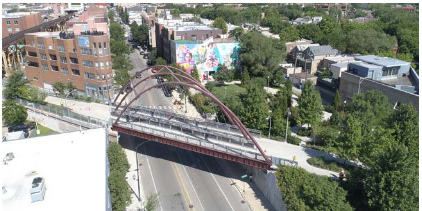
Figure 3.3: Milwaukee 606 Trail Bridge, Chicago, IL
