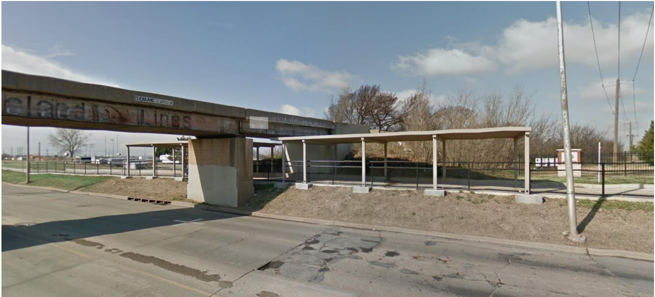
Figure 7 – Non-structural underpass covering for BNSF Crossing on the Will Rogers Trail
