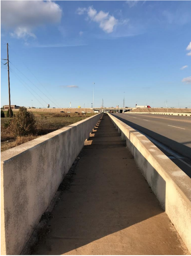
Location 9 – The S. Eastern Avenue bridge over the Oklahoma River will be reconfigured to accommodate the trail passing on the west side
