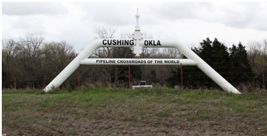
Figure 4-1. Pipeline Landmark in Cushing, OK
