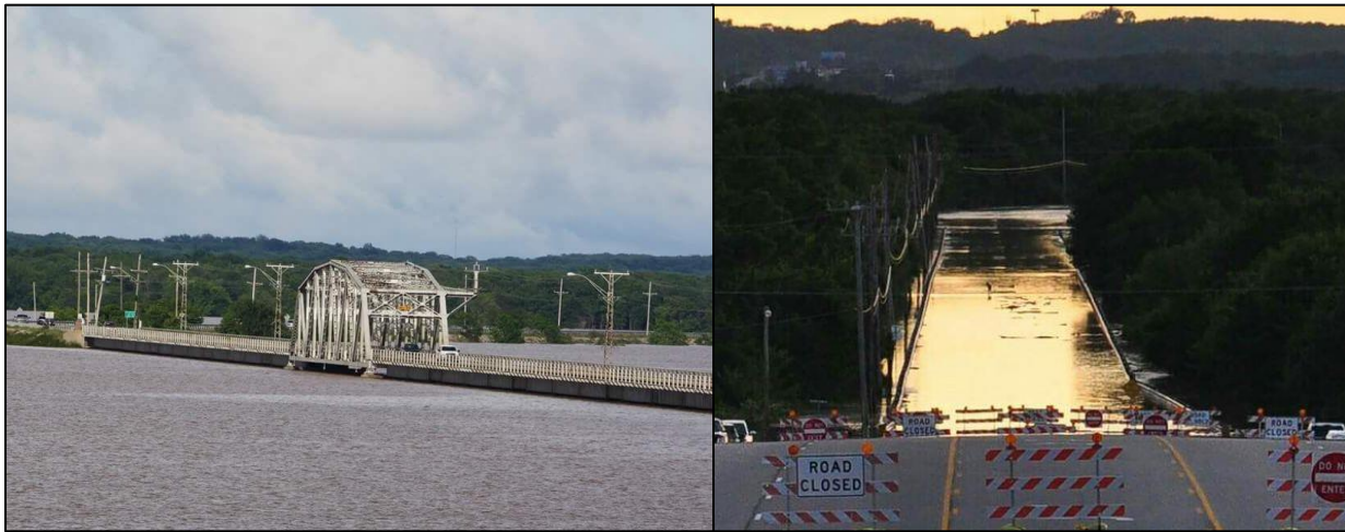
Figure 4: Roosevelt Bridge Flooding, 2015
