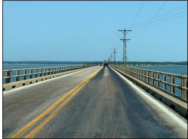
Figure 2: Roosevelt Bridge Narrow Deck Width
