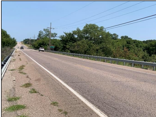
Photo 11: Segment 4 (End) - Looking East
