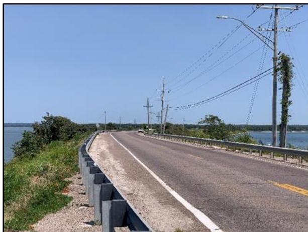
Photo 7: Lake Causeway - Looking East
