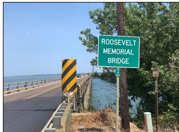
Photo 6: West Approach Looking East
