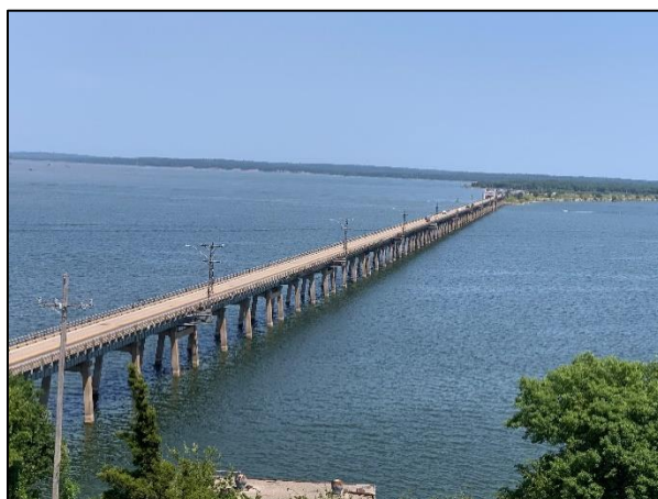
Photo 5: Roosevelt Memorial Bridge – Looking Northeast
