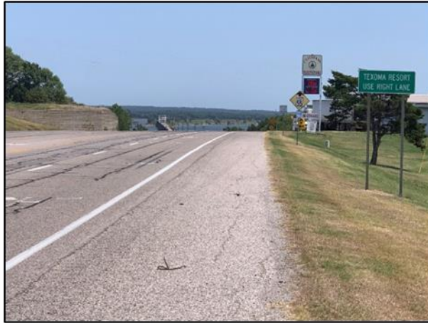
Photo 3: State Park Road Looking East
