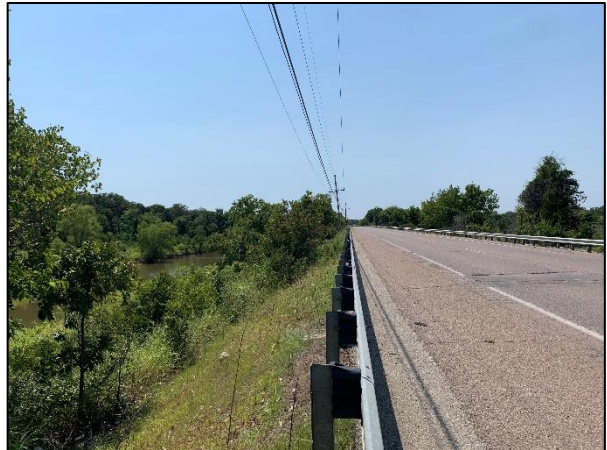
Photo 12: Segment 4 (End) - Looking West
