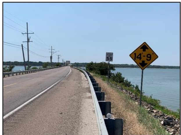
Photo 8: Lake Causeway - Looking West
