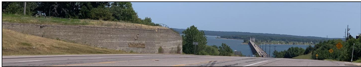
Photo 19: Existing Retaining Wall
