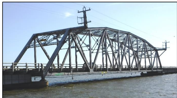
Photo 18: Bridge Warren Through-Truss
