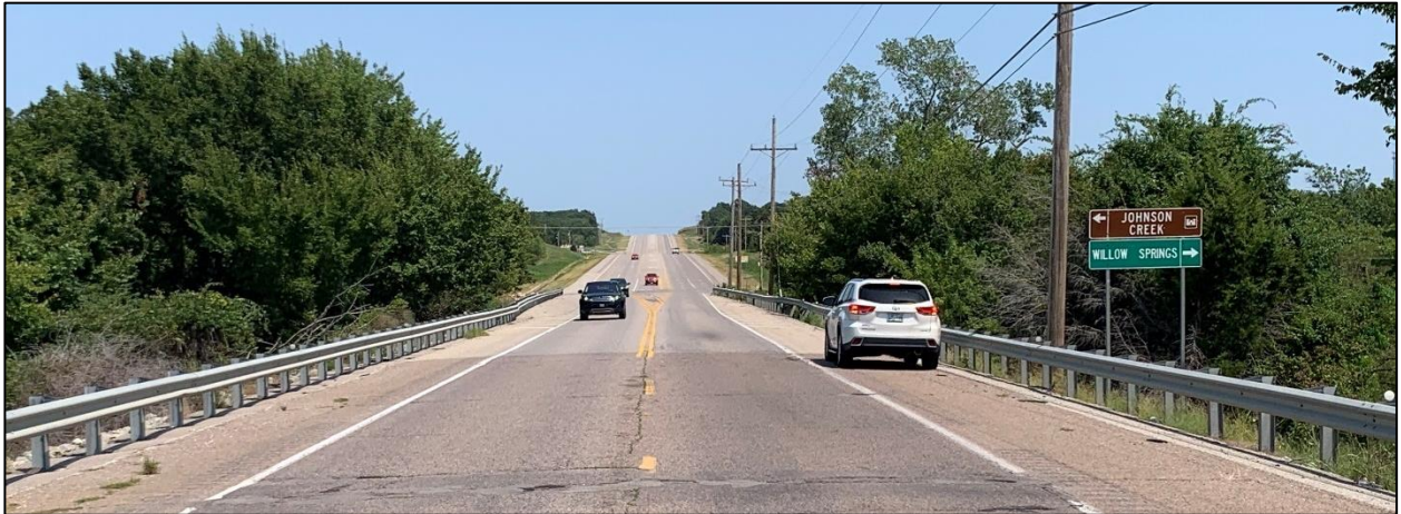
Photo 13: Lake Causeway - Looking East
