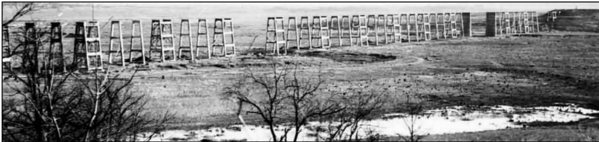
Photo 15: Roosevelt Memorial Bridge - Construction
