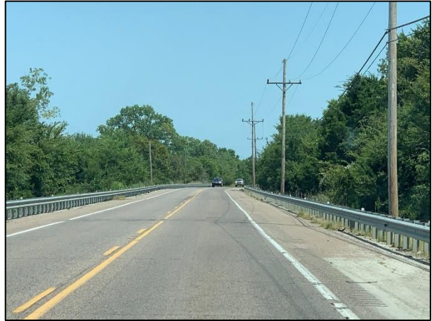
Photo 10: Segment 4 Begin - Looking East
