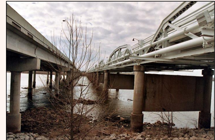
Jenks Pedestrian Bridge, OK
