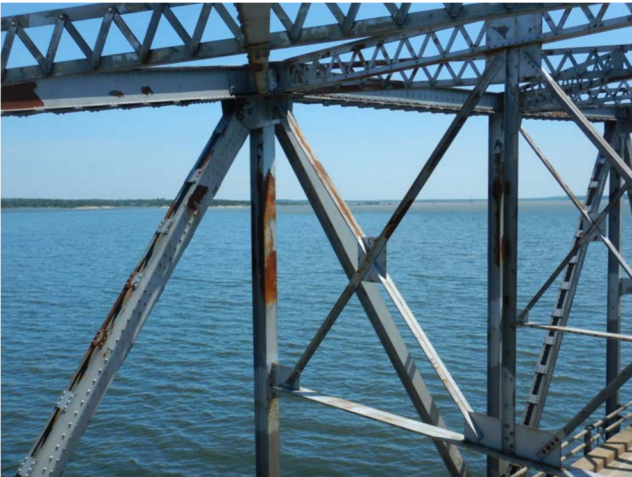
Photo 8: Typical Condition of Truss Sway Bracing (Previously Replaced)
