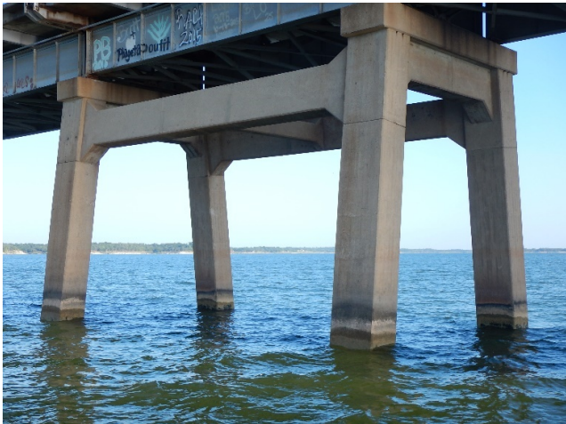
Photo 19: Typical Condition of Substructure (Tower Shown, Bent Similar)
