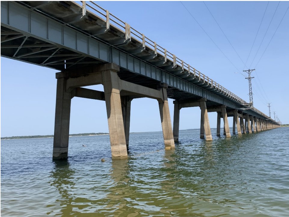
Photo 2: Roosevelt Memorial Bridge, Elevation
