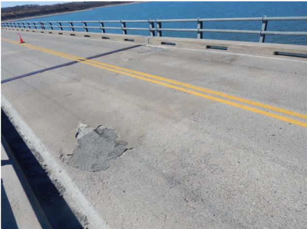
Photo 5: Typical Condition of Deck Slab
