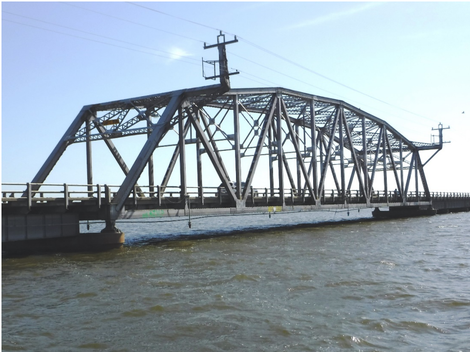
Photo 4: Truss Span, Elevation
