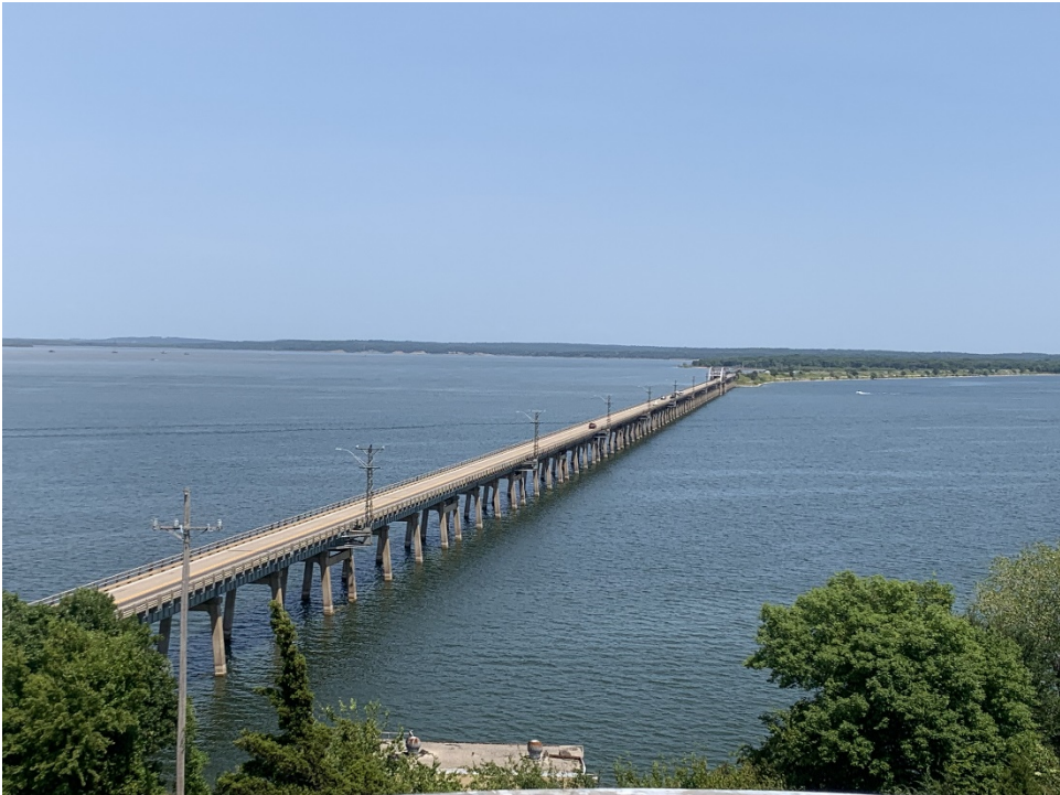
Photo 1: Roosevelt Memorial Bridge, Overall
