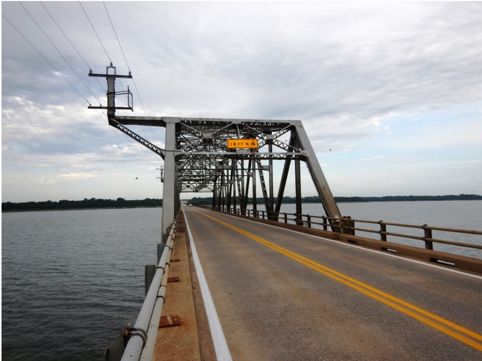
Photo 3: Truss Span, Approach
