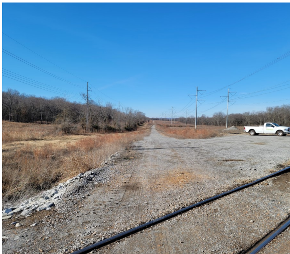
17. Point 5 looking to the east
