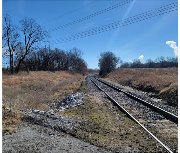
20. Point 5 looking to the north along the railroad.
