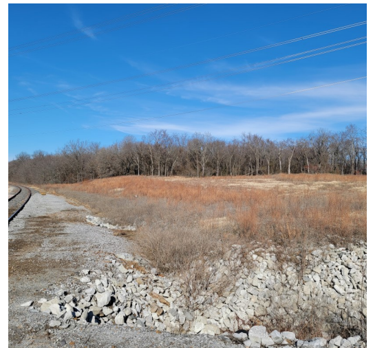
18. Point 5 looking to the north along the railroad
