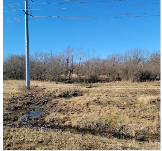
16. Point 4 looking to the west.
