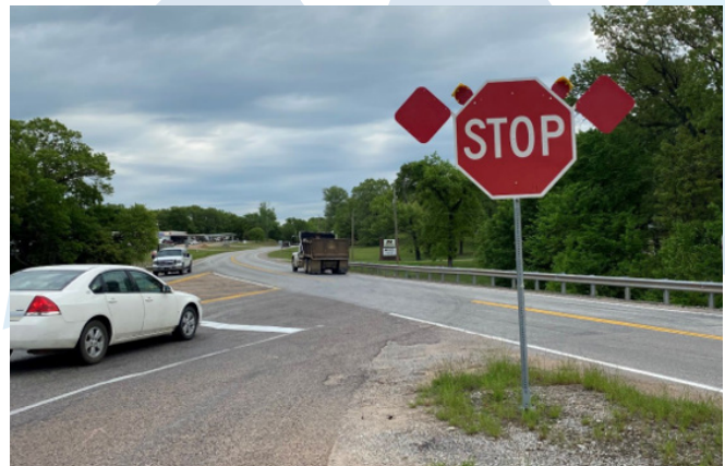
Figure 4: Stop Sign with newly installed red flags and flashing beacon on the sign (ODOT)
