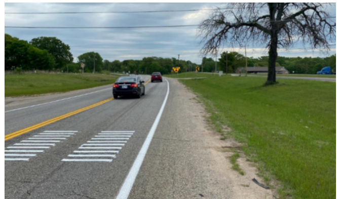
Figure 2: ODOT installed transverse rumble strips on eastbound SH-22 before the Advance Stop Ahead sign (ODOT)
