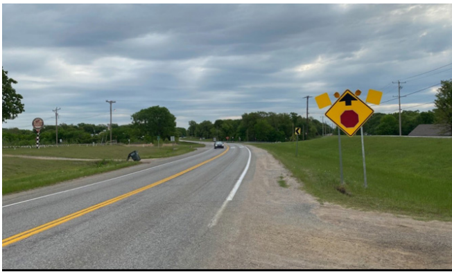
Figure 1: Eastbound view of flashing beacons and flags (Photo courtesy of ODOT)
