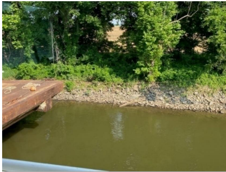
Existing Deadman Anchor wire at Oakley's Terminal Muskogee
