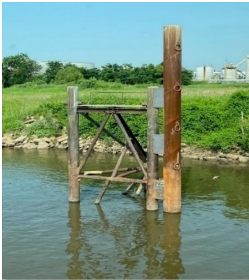
Existing Dolphin at the Port of Muskogee
