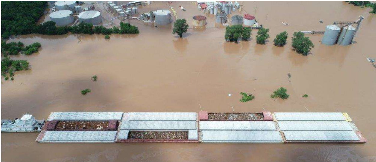
Figure 4. Underwater for nearly two weeks, barges at Port Muskogee broke loose and damaged downstream infrastructure, portions of the dock and wharf collapsed, electrical systems stopped working, and water flushed out sediment beneath railways, rendering them unusable.
