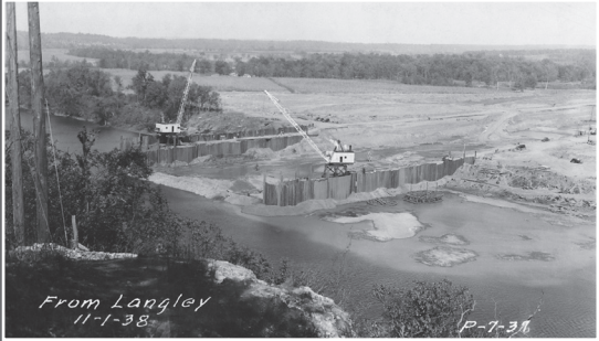
First concrete pour started in 1938
