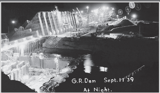
24-hour continuous pour continued for 20 months
