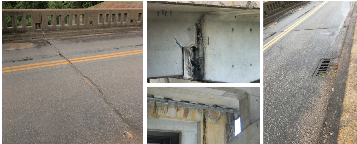
Example Bridge Conditions
