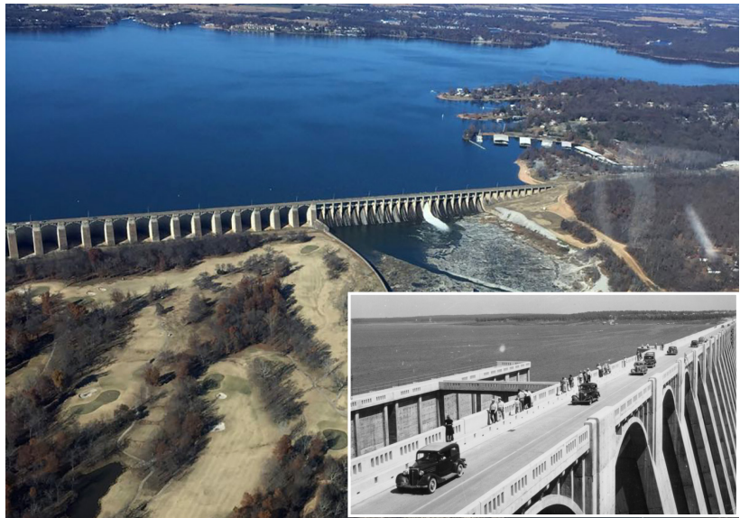
Aerial of roadway, spillway, Grand Lake
