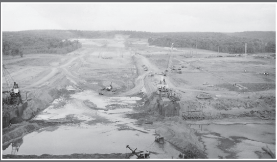
Preparation of the site started in 1937
