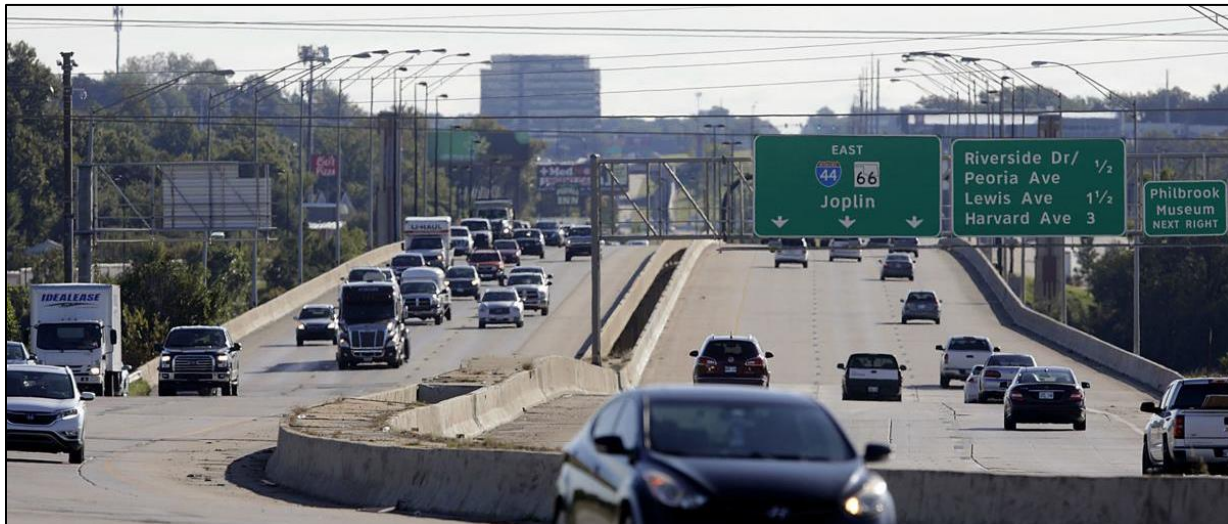
Figure 4: I-44 Bridge over the Arkansas River
