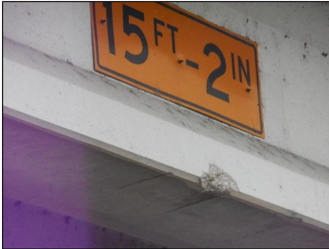
Figure 15: (L) I-44 over Elwood Avenue, Insufficient Clearance and Vehicle Damage, (R) Poor Pavement Condition on I-44
