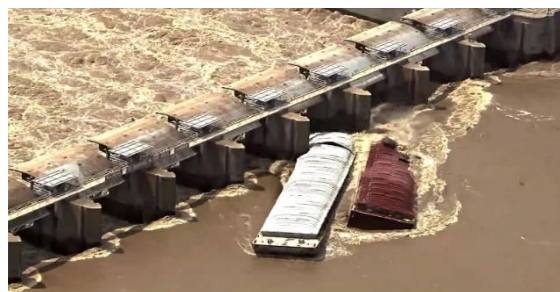
MKARNS dam near Webbers Falls Source: The Waterways Journal
