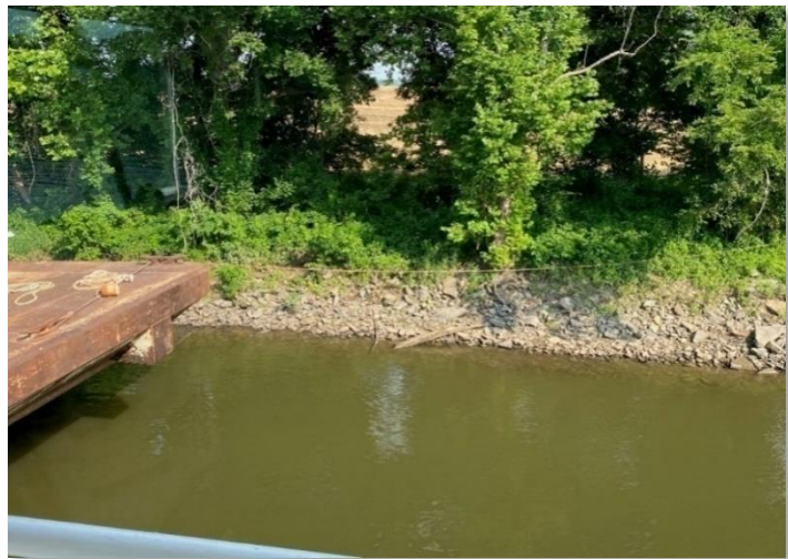
Existing Deadman Anchor wire at Oakley's Terminal Muskogee
