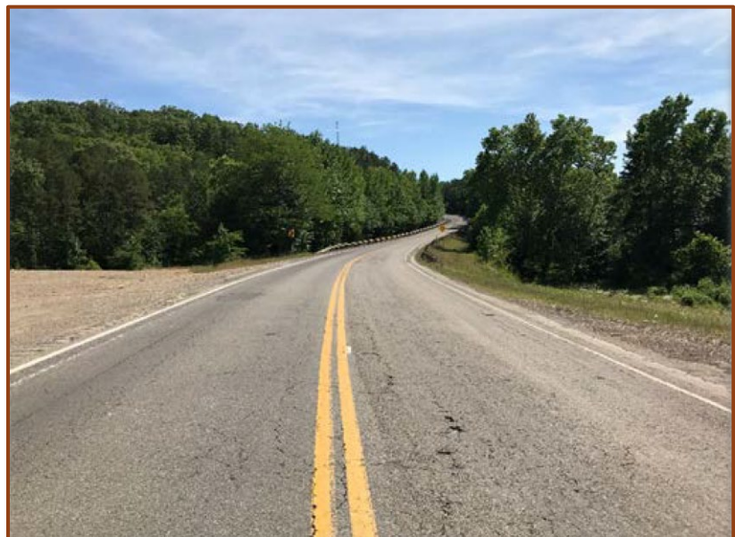
Figure 9. U.S. Route 259 North of Stevens Gap Road
