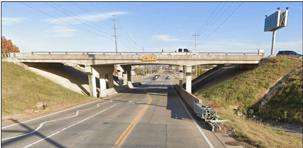
Figure 4: W. 81st Street under US-75 (facing east)
