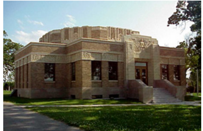
Figure 25: Tulsa Fire Alarm Building. Photo: David Stapleton
