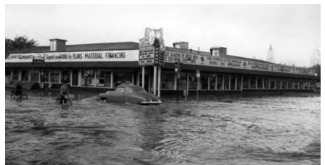
Figure 10: Storm water flooding the intersection by Hanna Hardware & Lumber on the southwest corner of 3rd & Peoria, circa 1952. Photo: Beryl Ford Collection
