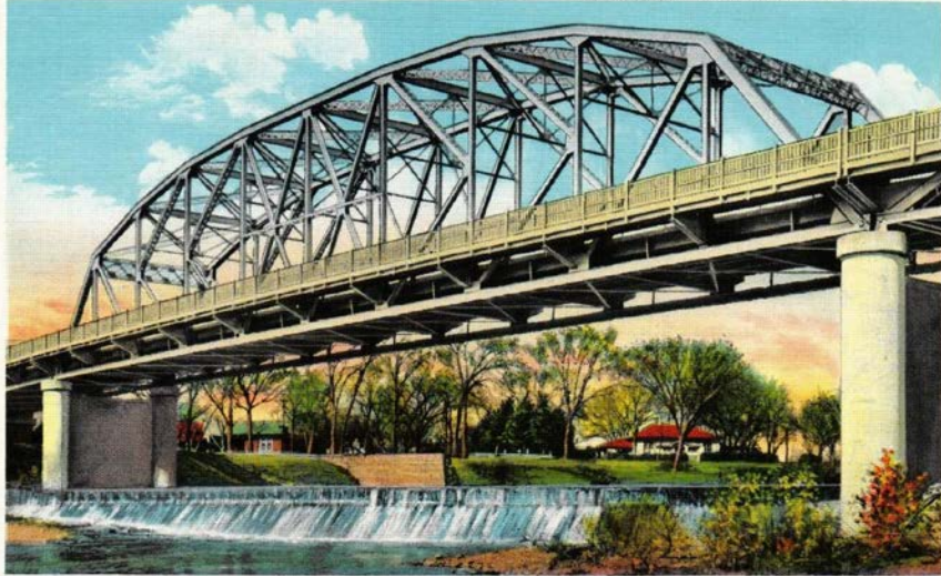
Caney River Bridge, Bartlesville, Okla.
