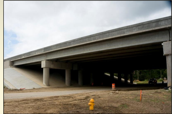
Example of a Prestressed Concrete Beam Bridge
