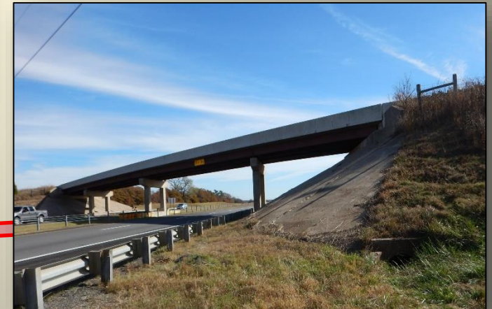
SE 59 th St. – Steel Beam Span Bridge
