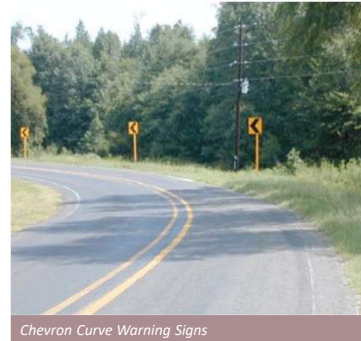
Chevron Curve Warning Signs
