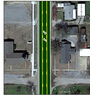
Future 3-Lane Section in Minco
