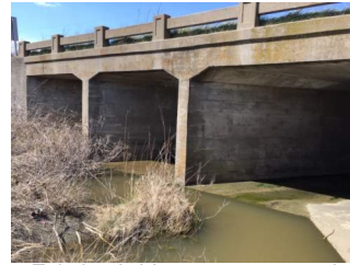
Existing bridge over unnamed tributary to Rock Creek
