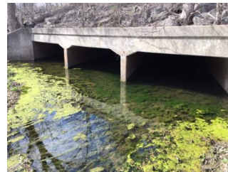
Existing bridge over unnamed tributary to Neosho River
