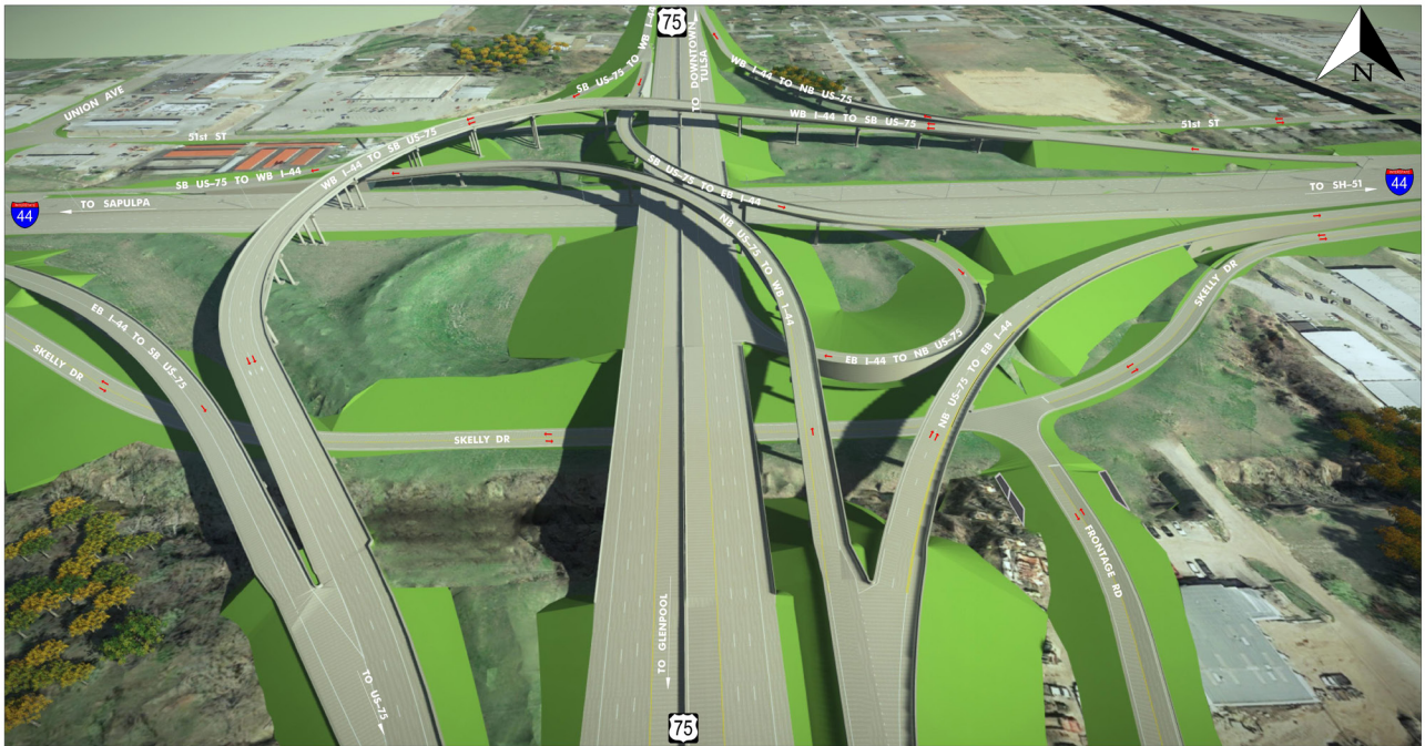
I-44/US-75 INTERCHANGE LOOKING NORTH
