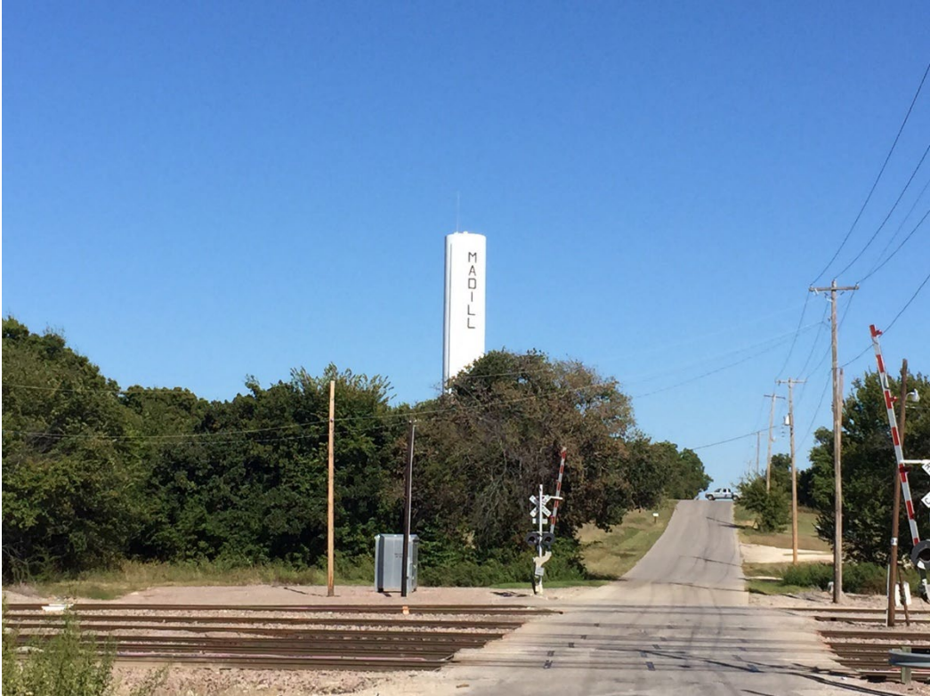
Photo 3: Water tower and railroad track crossing
