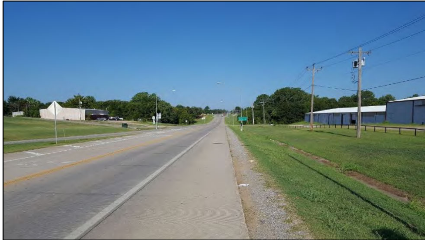
Photo 1 – Typical view of the existing US-70 in Madill. View from northwest project terminus, facing west.
