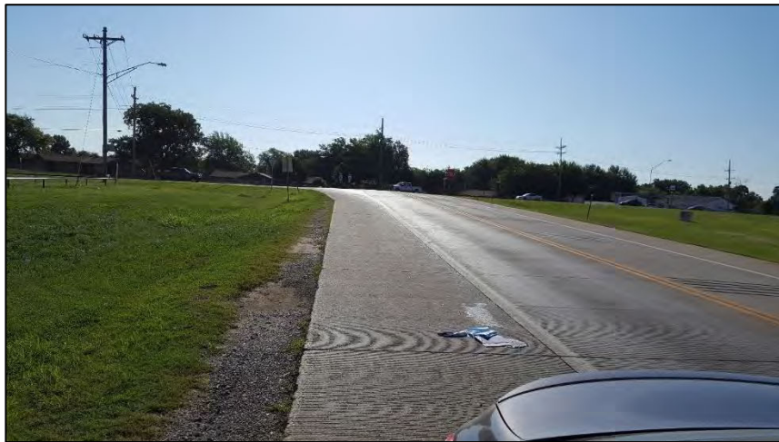
Photo 2 – Typical view of the ROW for existing US-70 in Madill. View from northwest project terminus, facing east.
