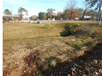
Photo: Developed area adjacent to project area
