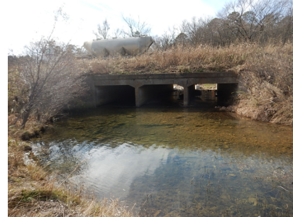
Photo: Crossing of US-259 over Yashau Creek
