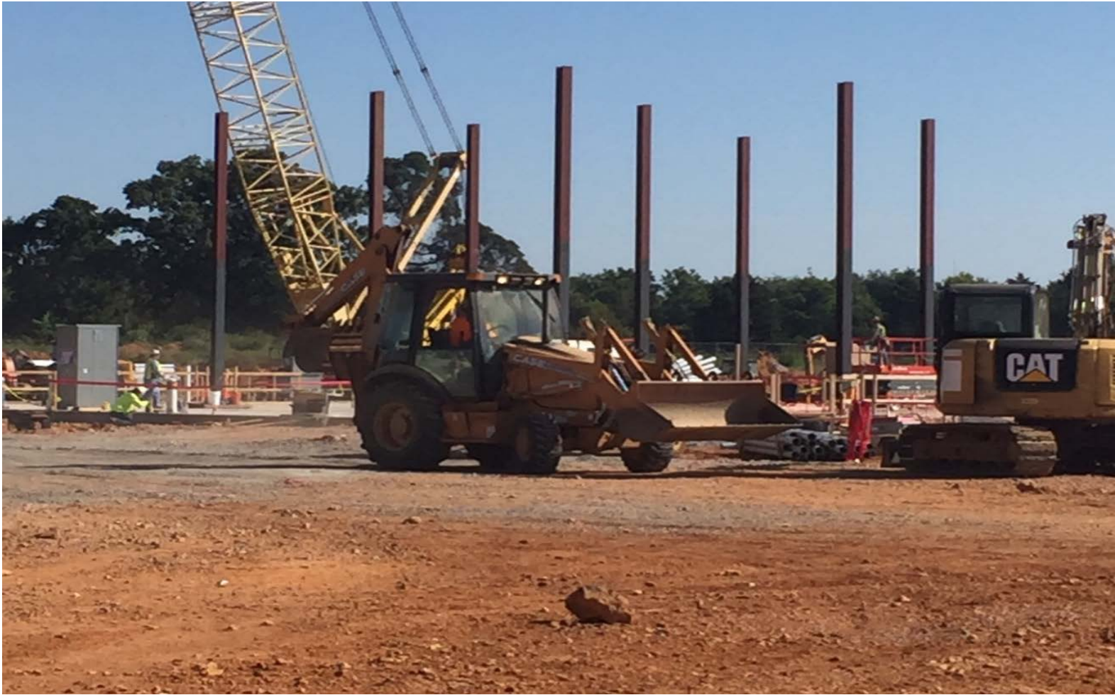
Superstructure Steel Going Up (September 2017)
