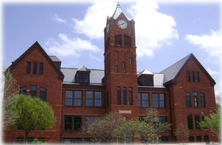
Old North Building, University of Central Oklahoma
